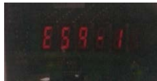
Figure 5. Error code shown on remote controller of VRV system
