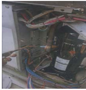
Figure 8. The replacement work on VRV compressor in Building 37
