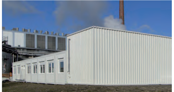
Garage for a company fire brigade
