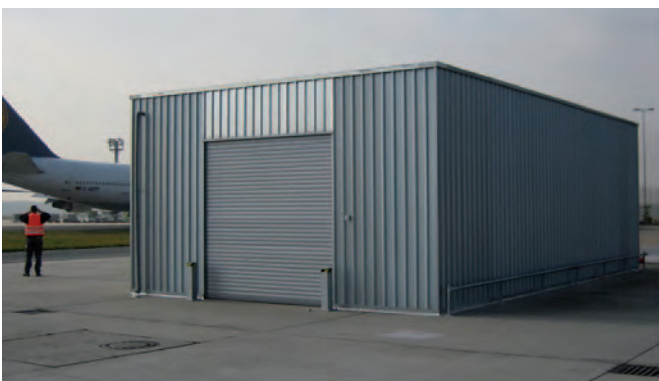
Materials store on the airfield
