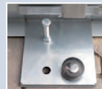
Ground anchorage with ground nails, without foundation
