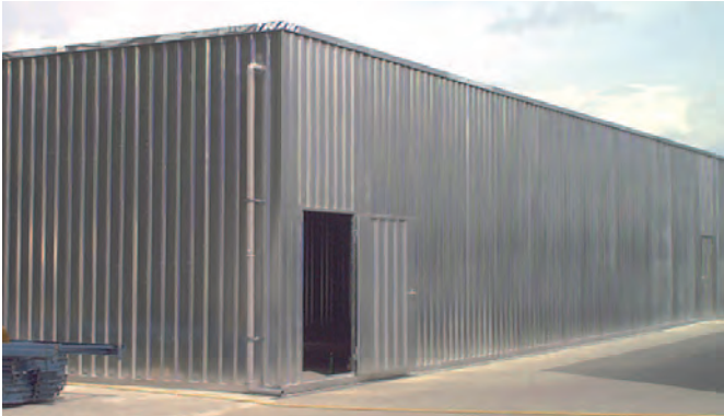
Warehouse for a wholesale business
