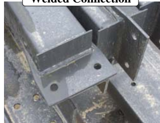
Welded Connection
