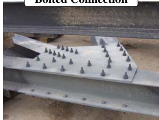
Bolted Connection
