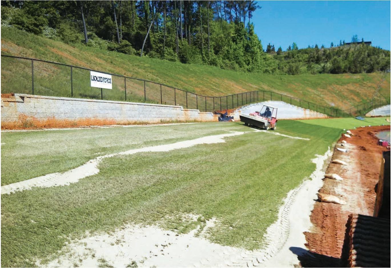
PHOTO 5 Grooming the binder material infill into the turf.
