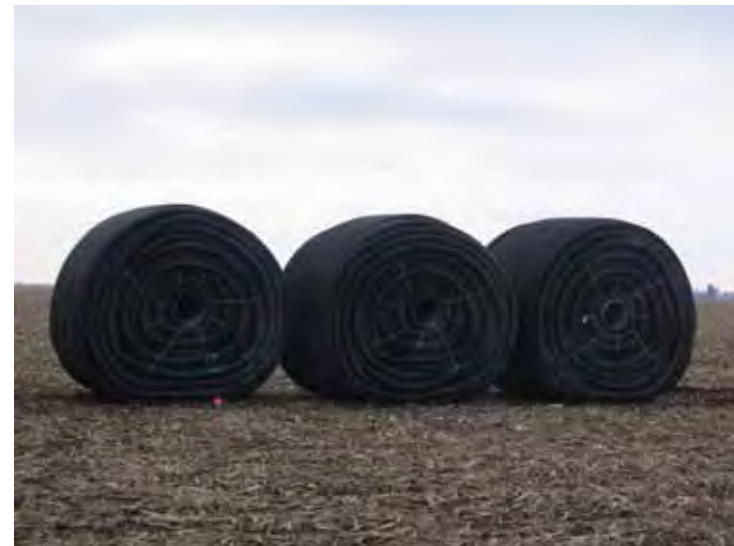
Corrugated polyethylene tile waiting to be installed.
