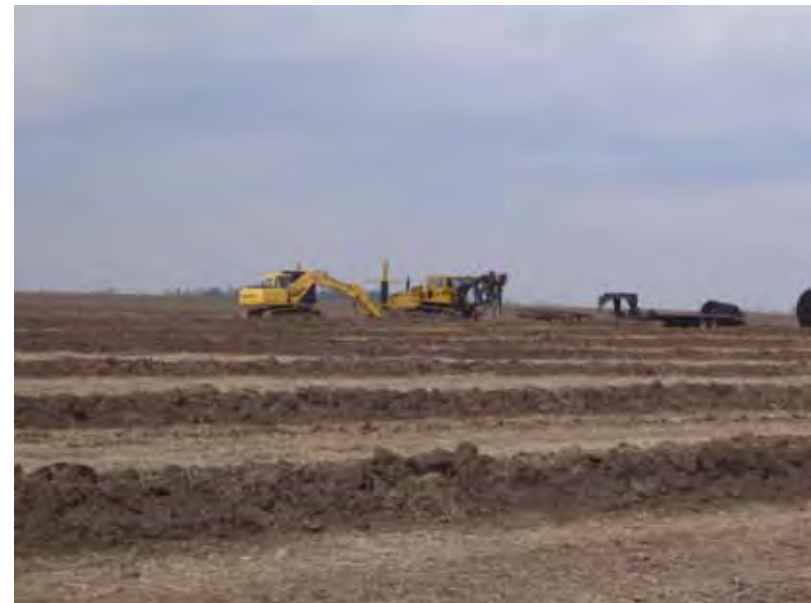
Field with drainage tile installed using a trenchless tile machine.
