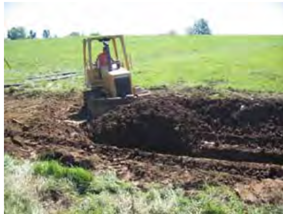
Small bulldozer backfilling a tile trench.
