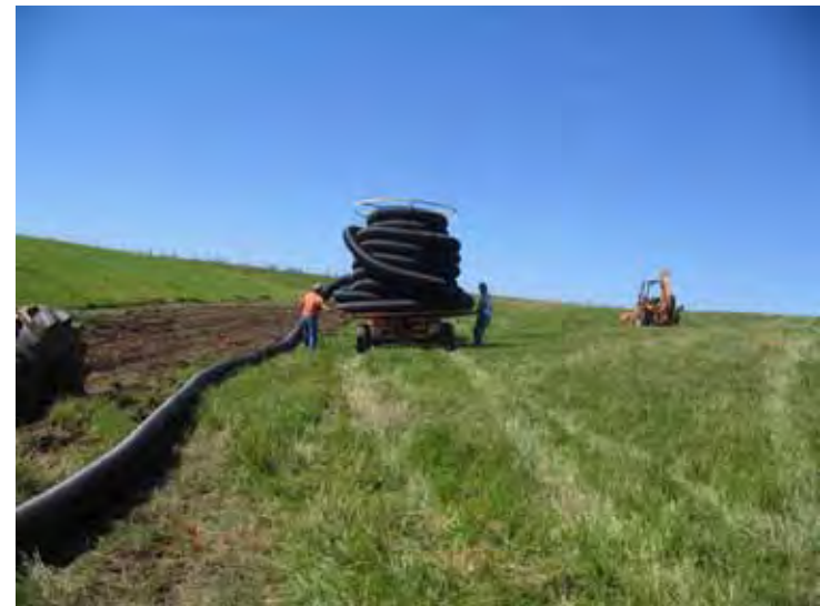
Corrugated polyethylene tile being unrolled for installation.
