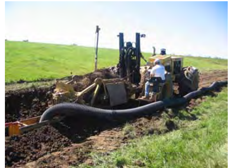
Corrugated plastic tubing being installed by a trencher type tile machine.
