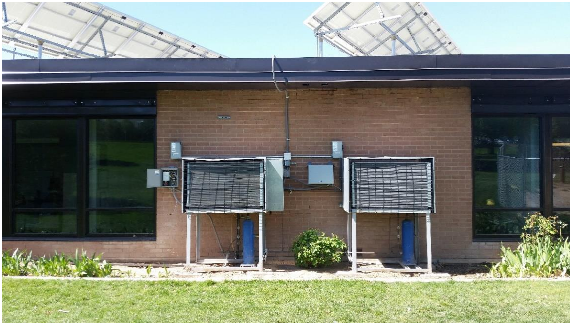
Figure 2.3. HVAC systems for the two thermosiphon arrays.
