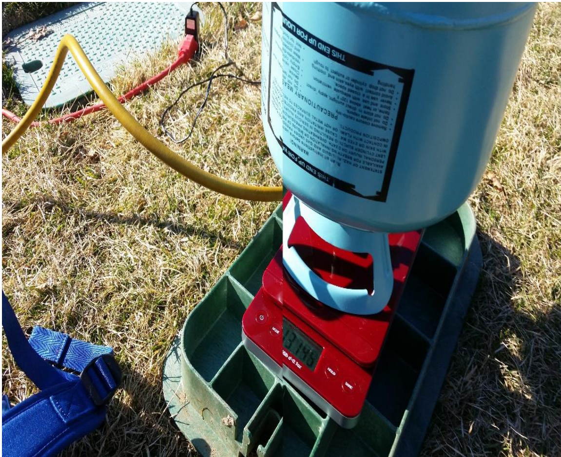
Figure 2.7. Charging the thermosiphons with R-134a.
