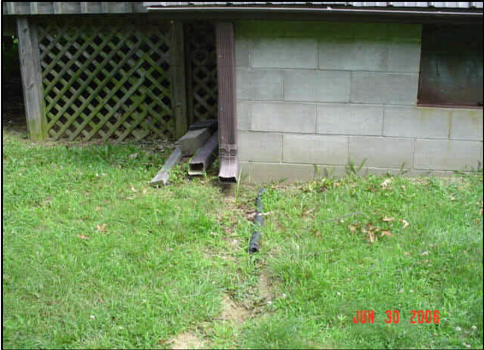
Small area of past water ponding from gutter runoff and sump pump discharge was observed near SW corner of the Subject's foundation.
