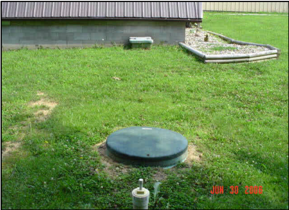
Subject's septic system was operating during the inspection and show no signs of failure, etc. This is an aeration type septic system common to the neighborhood where municipal sewage systems are un-available.
