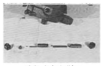
FIG. 36. Acceleration Valves
