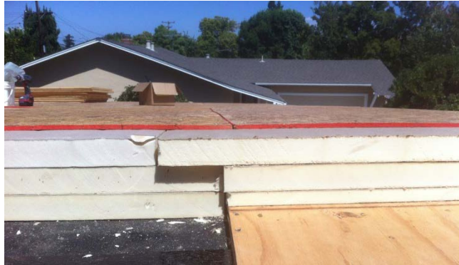
Figure 2. Six inches of roof deck insulation
