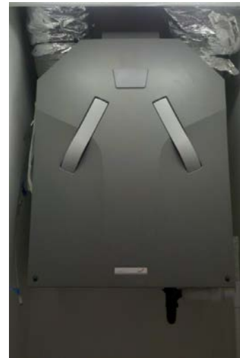
Figure 5. Zehnder ComfoAir HRV
