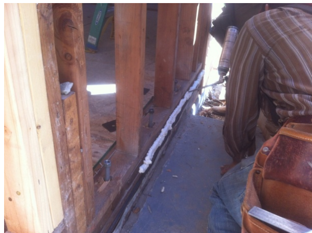
Figure 3. Applying spray foam
