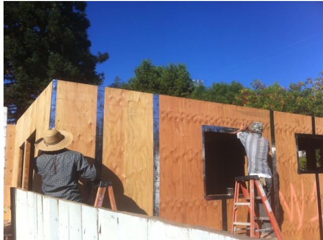
Figure 4. Taping of joints
