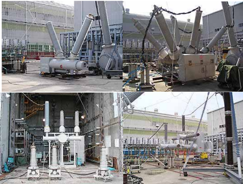
Gambar X. 18 Gambar-Gambar Short Circuit Breaking Tests
