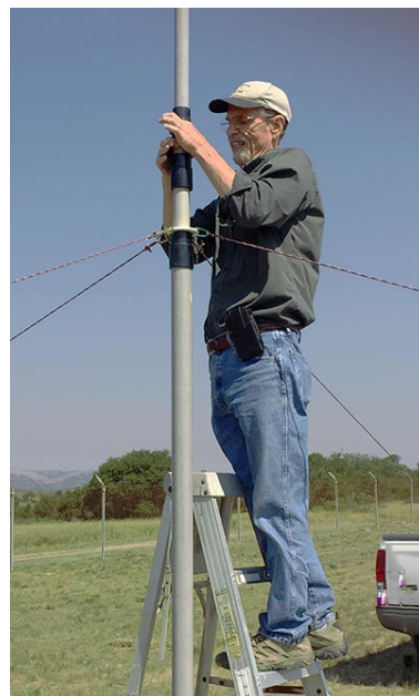
Figure 8: Dayle Good KK6HNS pushing up mast sections while helpers gently hold the top guys..
