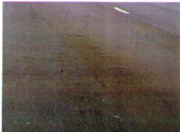
Figure 9 - Blisters forming on SAF layer
