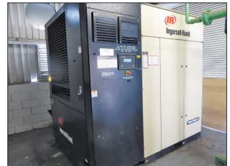
150-HP Ingersoll Rand Model IRN150H-CC Air Cooled Rotary Screw Air Compressor
