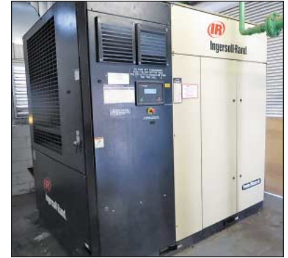
150-HP Ingersoll Rand Model IRN150H-CC Air Cooled Rotary Screw Air Compressor
