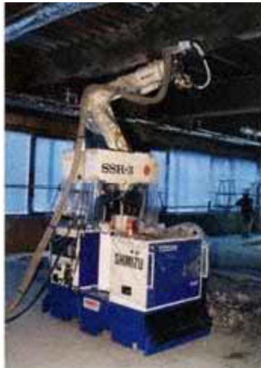
Figure 16. Fire-retardant spray coating robot [source: Shinko 2007].
