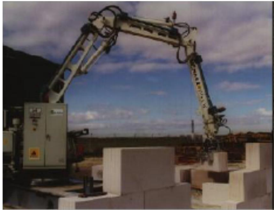
Figure 13. ROCCO project brick assembly robot [Source: Balaguer & Abderrahim 2008].
