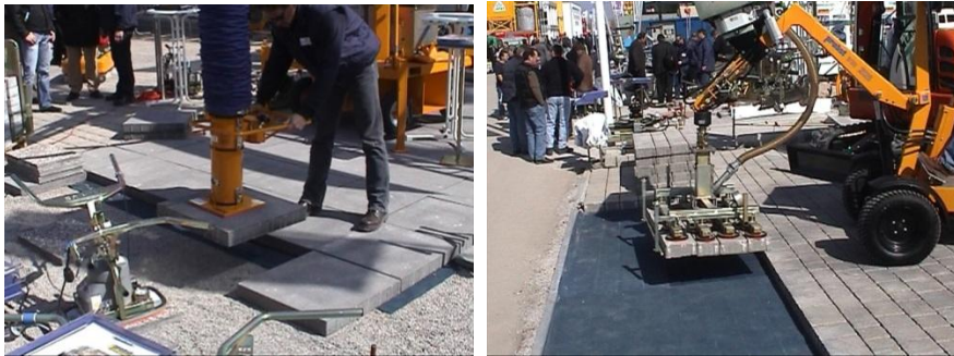
Figure 17. Slab installation machines (Courtesy by Hannu Koski).
