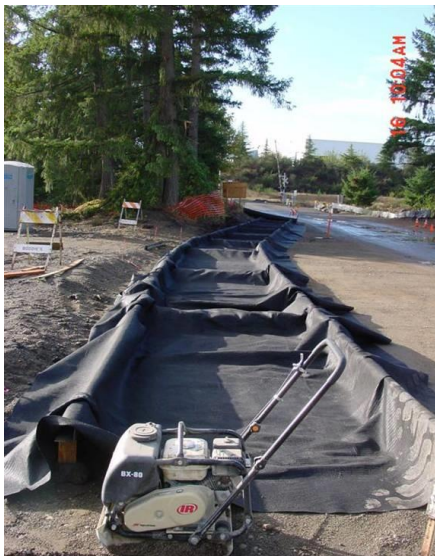
Figure 9: Line with Geotextile
