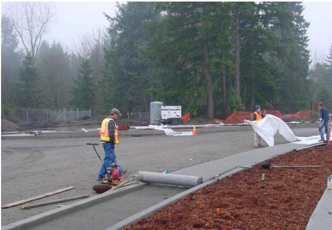
Figure 13: Place Second Lift of Pervious Concrete
