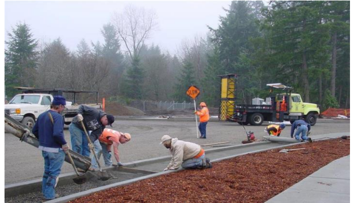
Figure 12: Place First Lift of Pervious Concrete
