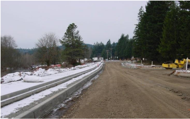
Figure 11: Backfill Drain Rock and Compact
