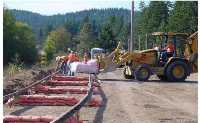
Figure 8: Excavate & Check Dams
