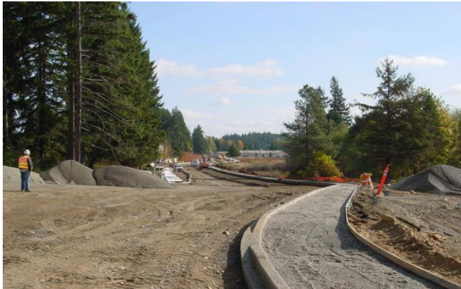
Figure 7: Sidewalk First & Outside Curb
