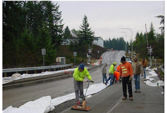
Figure 14: Screed, Roll, Compact, and Cover
