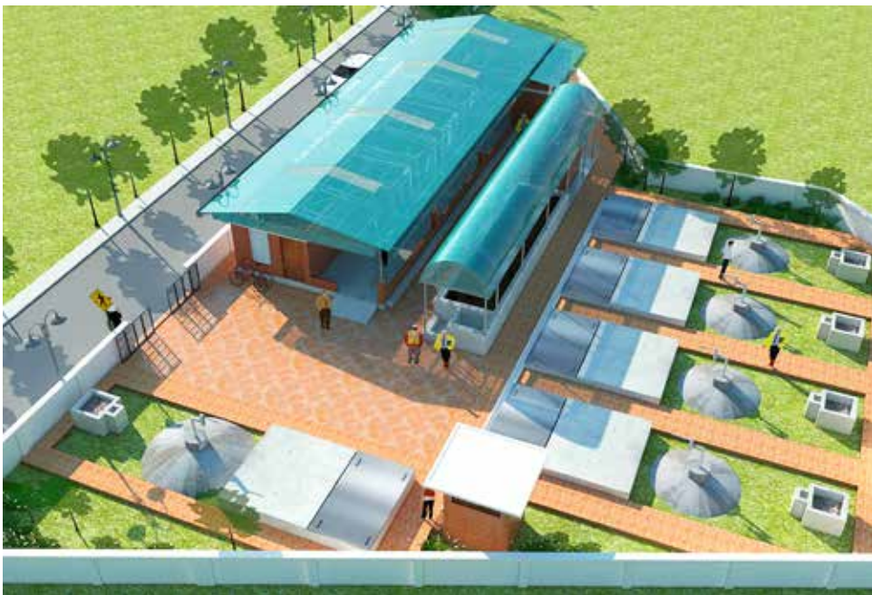
Figure 3.b. Plan of IRRC in Malang Regency, Indonesia (with compost plant, biogas plant, faecal sludge treatment plant, and trickling filter for waste water treatment plant).
