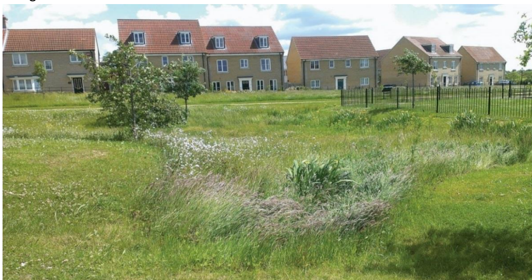
Figure 5: Detention basin with amenity planting and easy access for maintenance. A space that contributes to placemaking values by being welcoming, safe and pleasant. Source: The SuDS Manual C753
