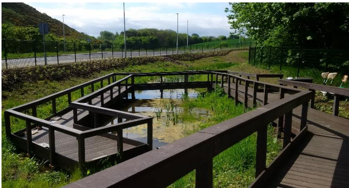
Figure 13: Roads and playing pitches drainage at Law Primary, Haddington Road, North Berwick, naturally regenerating with local species, and providing access for education via a boardwalk. Source: author's photo
