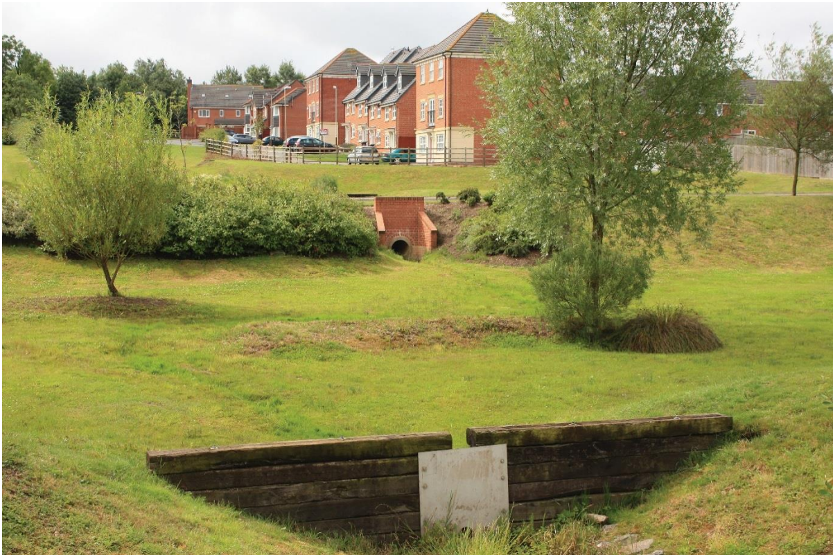
Figure 6: Detention basin providing water detention as well as usable attractive amenity space with raised areas for planting and a variety of side slope gradients, being adaptable and resource efficient. Source: The SuDS Manual C753
