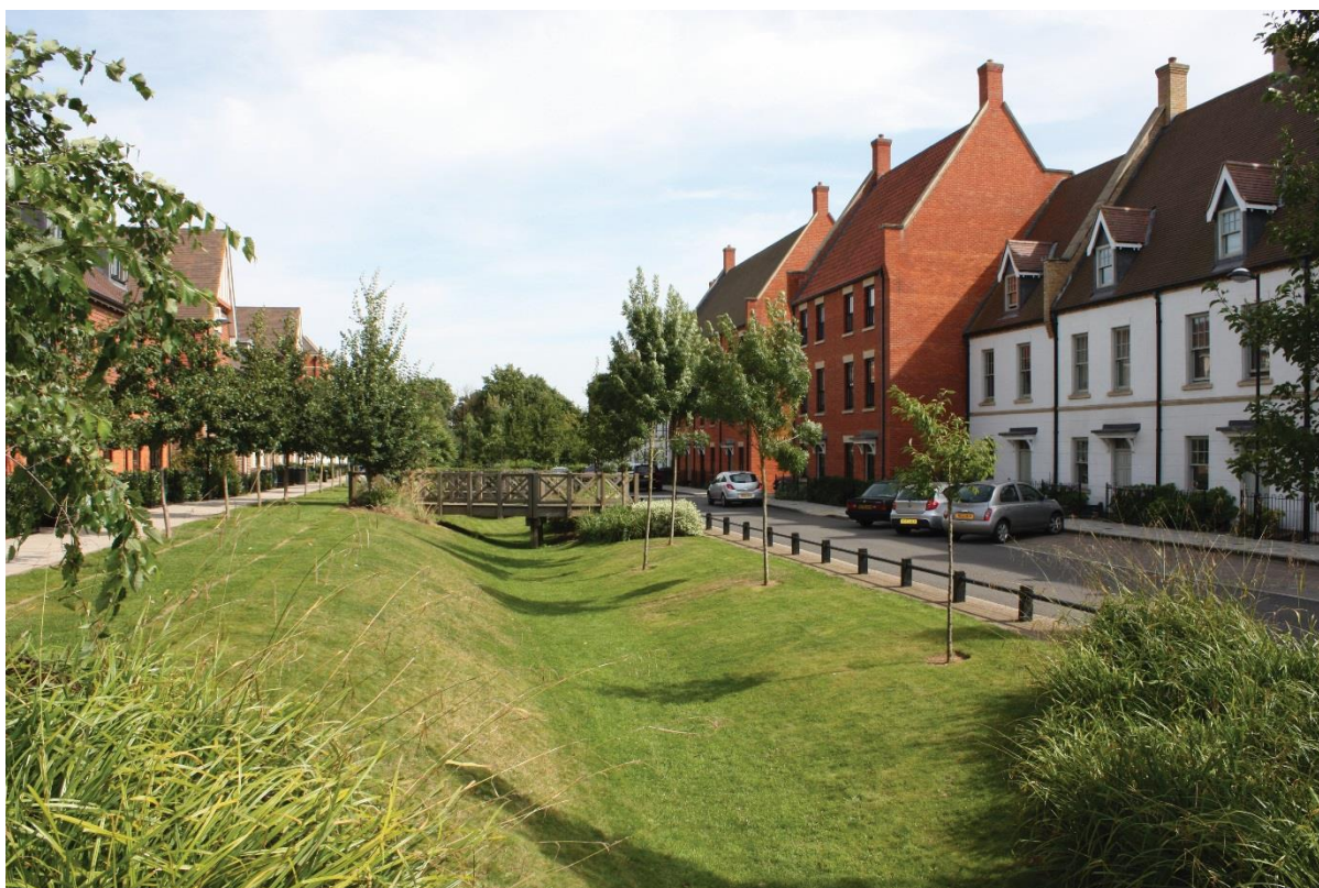
Figure 8: Shallow formal grassed swale wide and shallow enough to be cut by a ride-on mower. Note low fence to prevent vehicle over-run. Source: The SuDS Manual C753
