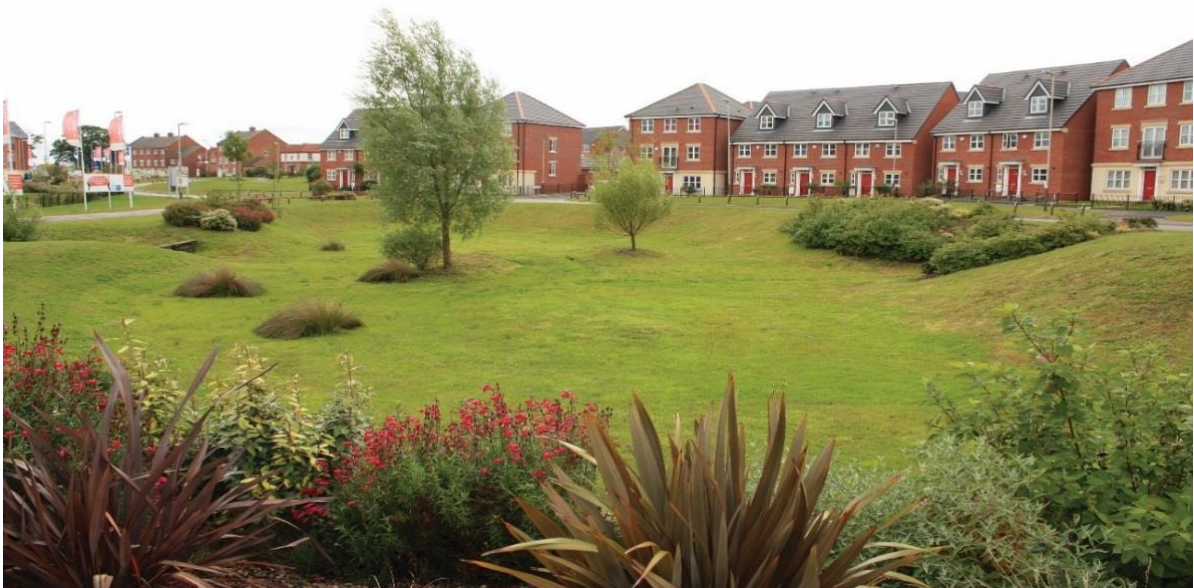
Figure 1: Detention basin providing water detention as well as usable attractive amenity space with a wide base and relatively shallow slopes. Source: The SuDS Manual C753
