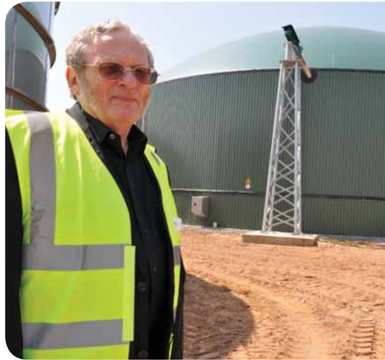
Cllr Becket outside the anaerobic digestion unit at Lower Reule
