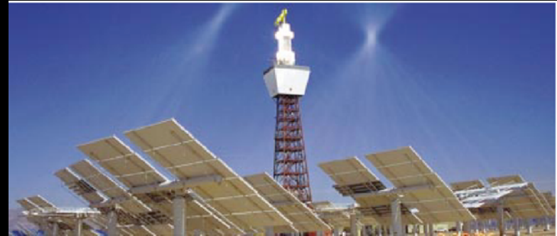
During daylight hours, 2000 mirrors at Solar Two track the sun and store its energy as heat in molten salt. This energy can then be used to generate electricity when needed, such as during periods of peak demand for power.
