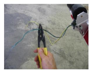
Cut the excess wire at the rear of the trailer leaving 12" exposed.
