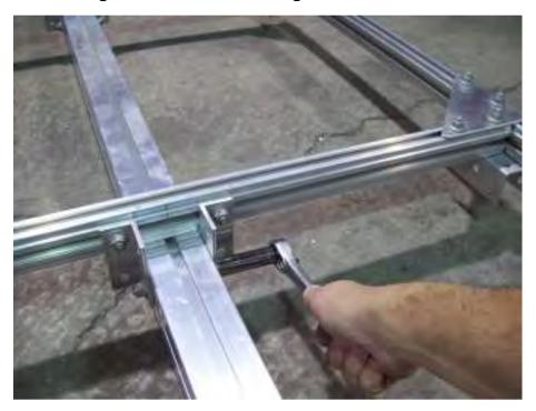
Once brackets are aligned with pencil marks tighten all nuts.
