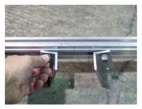
Install the angle brackets on the T-bolts, already in the cross members as shown.
