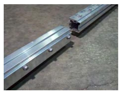
Lay the tongue sections end to end with the splice plates adjacent to each other.
