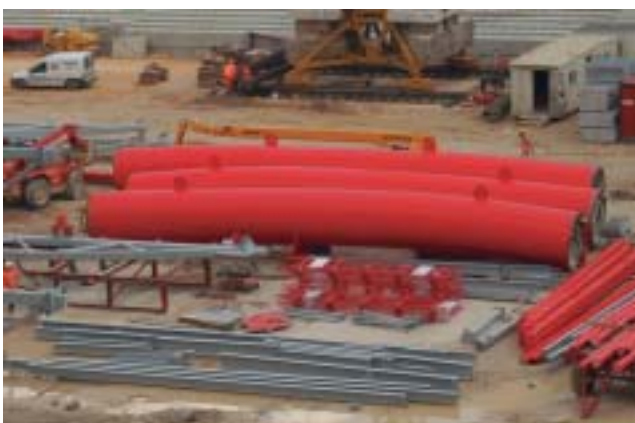
Figure 2. 24m long prefabricated arc sections waiting to be lifted in place.
