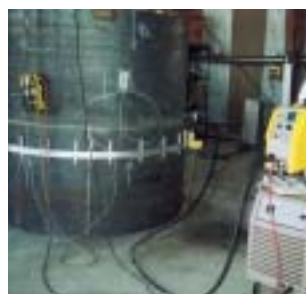
Figure 2. Set-up during welding procedure qualification.
