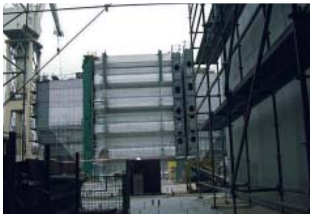
Figure 1. Corrugated bulkhead in the Bow Sun.
