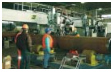
Figure 4. The submerged arc welding portal with two ESAB twin-arc heads.
