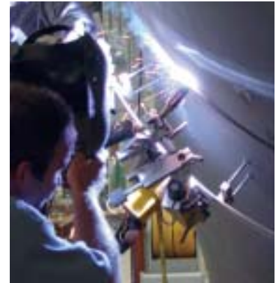
Figure 8. FCAW with FILARC PZ6113 and Railtrac FW 1000.
