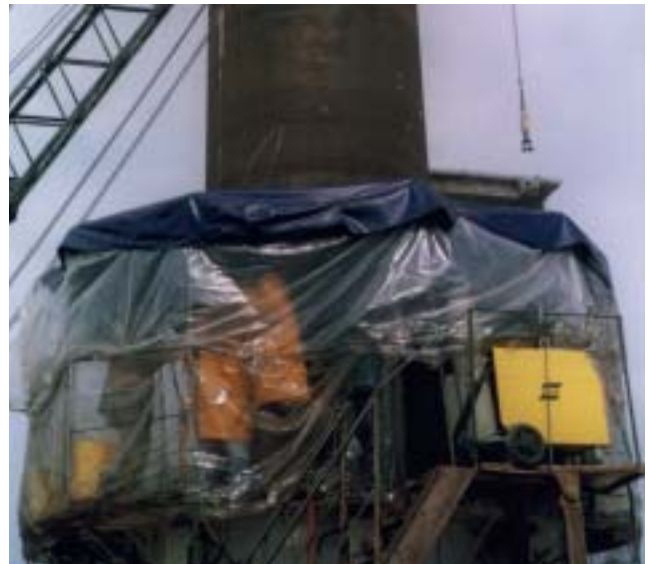
Figure 5. Welding station on site.
