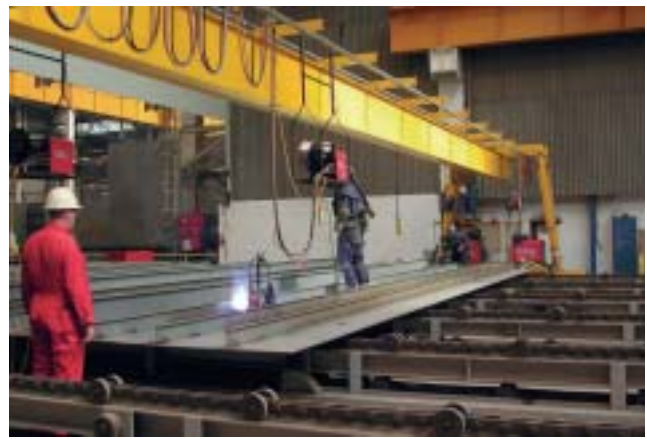
Figure 2. Primed bulk flats being welded with ESAB Tubrod 14.11.
