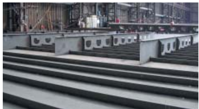
Figure 3. Tee stiffeners being assembled onto panel at Pt Clarence yard
