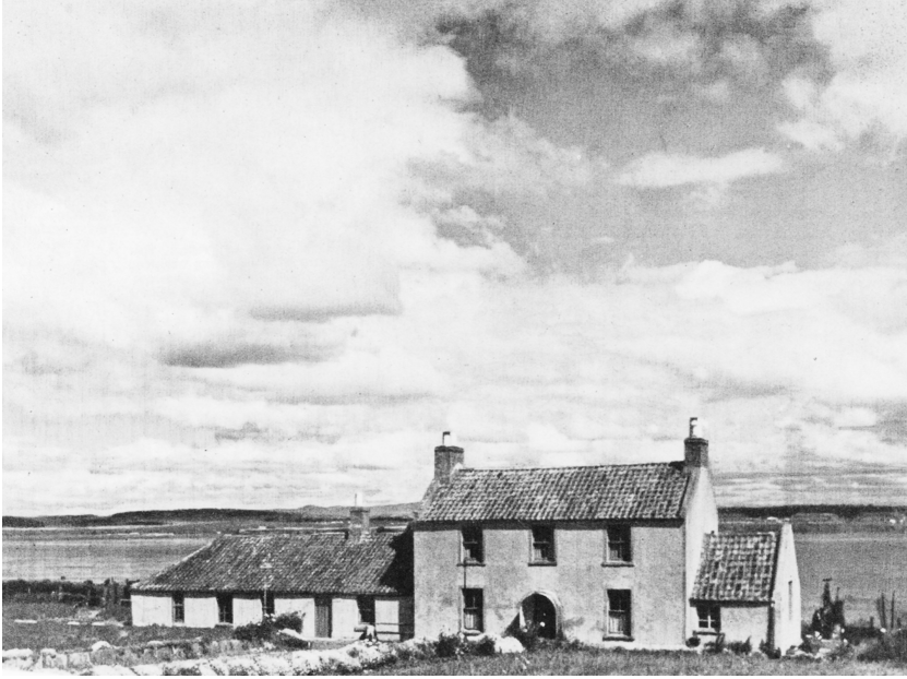
The cottage on Barrandale Island, before renovations and repainting, c.1960.
