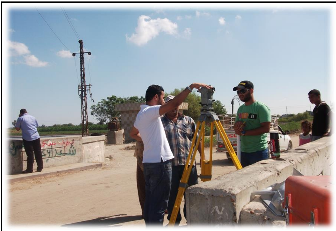
Photo 2: Land leveling at the village bridge.
