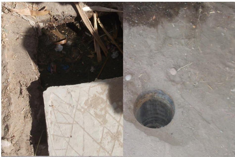
Photo 1: The common sewage disposal systems at the village
