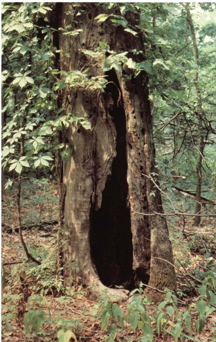
Figure 38.—Butt scar on sycamore and resulting decay.
