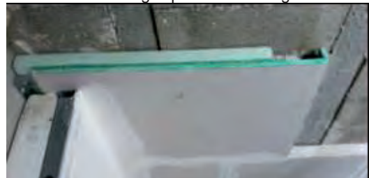
Figure 3: STB installed on-site – Thickness = 43 mm
