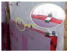
Figure 2 - Installation of VIP panel with Clip-on concept (W2) – S-shape clips.
