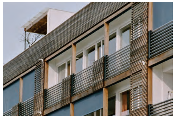
Picture 1: Slender south façade with VIP around the windows. The balconies are shading the windows and solar collectors are integrated in the railings.
