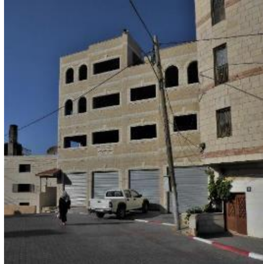
Image 27 Ramallah: building in construction in the old village; contemporary opening, far from the stone wall esthetic (photo RC)
