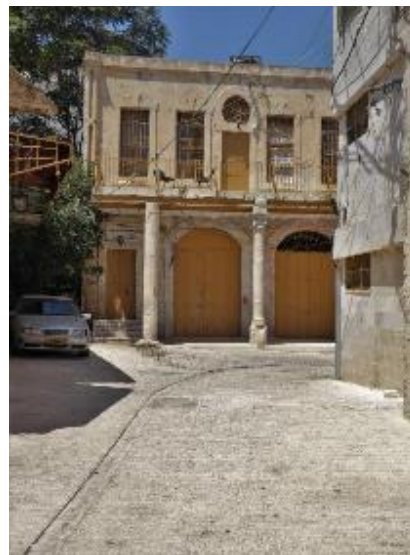
Image 23 Hebron: Historic-modern town-house and commerce, a mandate period building (photo RC).
