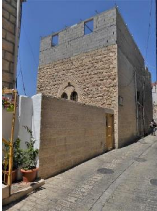
Image 7 Hebron: A restored building. Several kinds of stones in this building; undressed stones seen in the wall with arched window and new dressed stones (hadjar imsamsm) facing the street. At the upper level, we can see some concrete blocks .... (photo RC)
