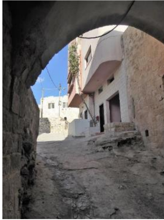
Image 6 Sanur: arched passageway inside old quarter, structural stone walls, cladded walls and plastered ones compose the contemporary townscape (photo RC)
