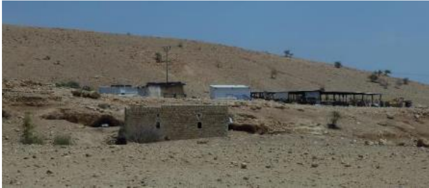
Image 46 al-'Auja: mixed building material: stone, tent and sheet metal (photo RC).
