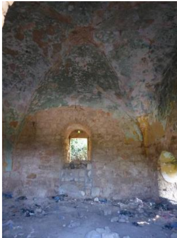
Image 15 Birzeit compound: Cross vaults ending with pointed vault interior traditional hall
