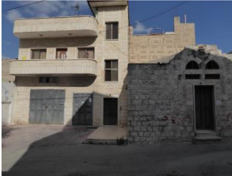
Image 1 'Arraba: Late Ottoman- early 20th century house and a recent one in concrete beams and dressed stones with wide openings on the front (photo RC)
