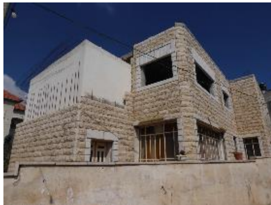
Image 26 Kafr Malek: Concrete and iron reinforced masonry (photo RC).
