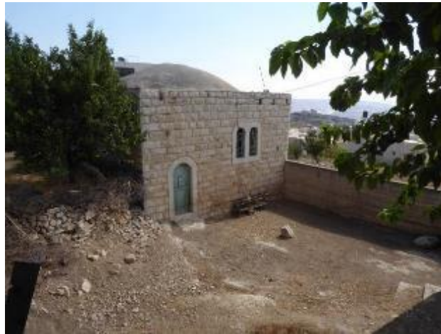
Image 13 Kafr Malek: Traditional independent Peasant/Fallāḥ house “end of the 19 th –beginning of the 20 th century.” Note the dome instead of flat surface (photo RC).
