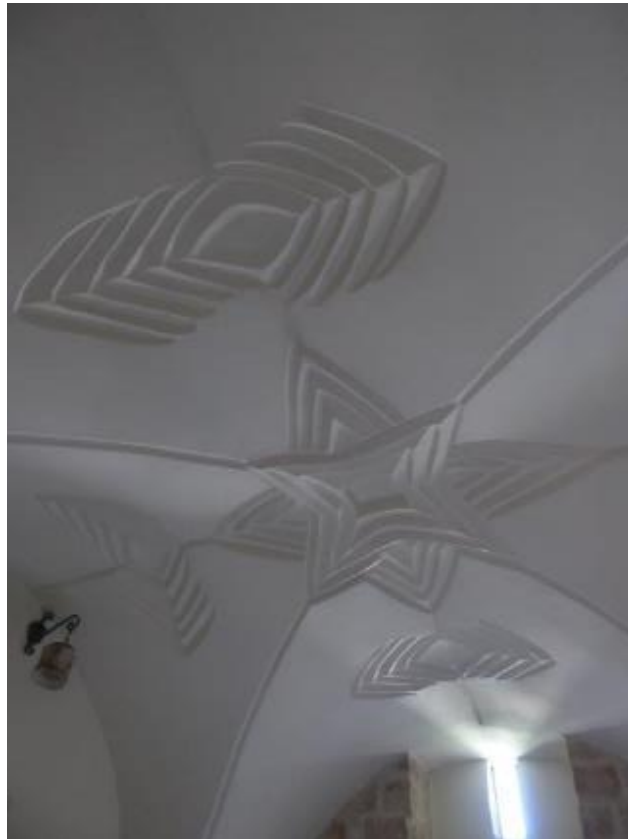
Image 11 Nablus Old City: plaster decoration. Cross vaults in "Arafat Soap Factory".
