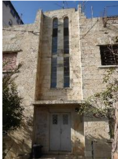
Image 22 Ramallah: modern openings in an independent house (photo RC).
