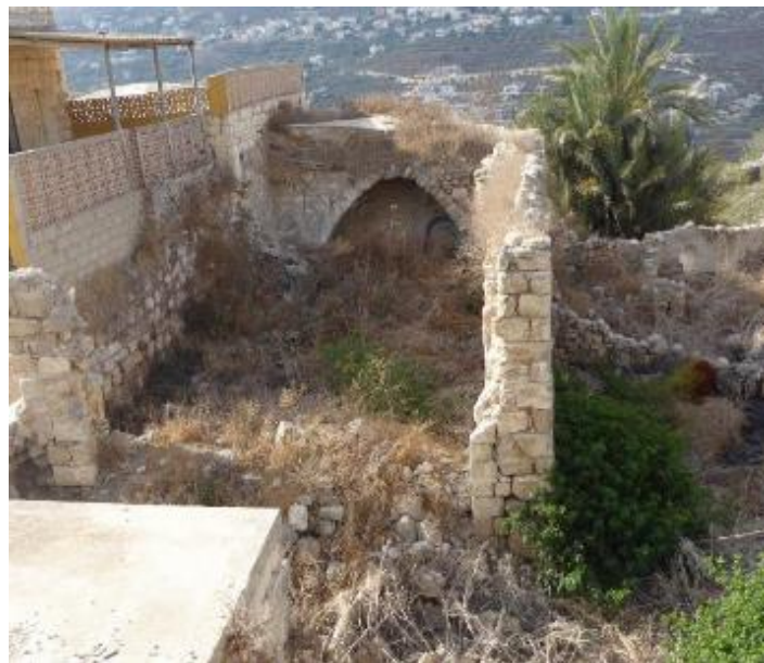
Image 8 Sebastia: ruins of an ancient traditional vault hall (usually the roof of such kind of these halls called djamalou - photo RC).
