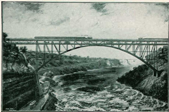
SINGLE ARCH DOUBLE TRACK STEEL BRIDGE OVER NIAGARA RIVER.
