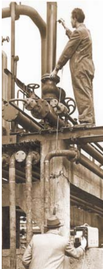
Wall thickness measurement: two are better than one.
