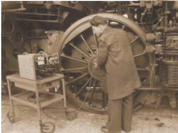
top: Weld testing
