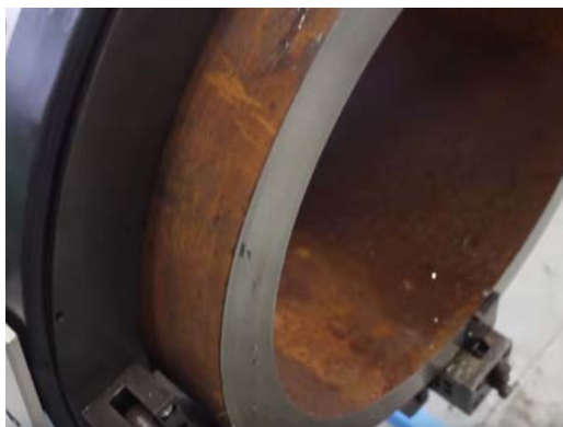
Pipe cold cutting
