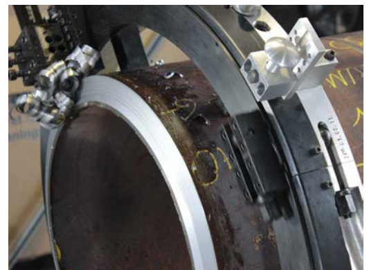
Pipe cutting and beveling
