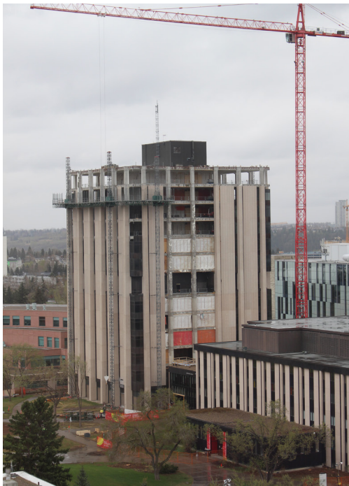
The former home of the GSA, MacKimmie Tower under construction.
