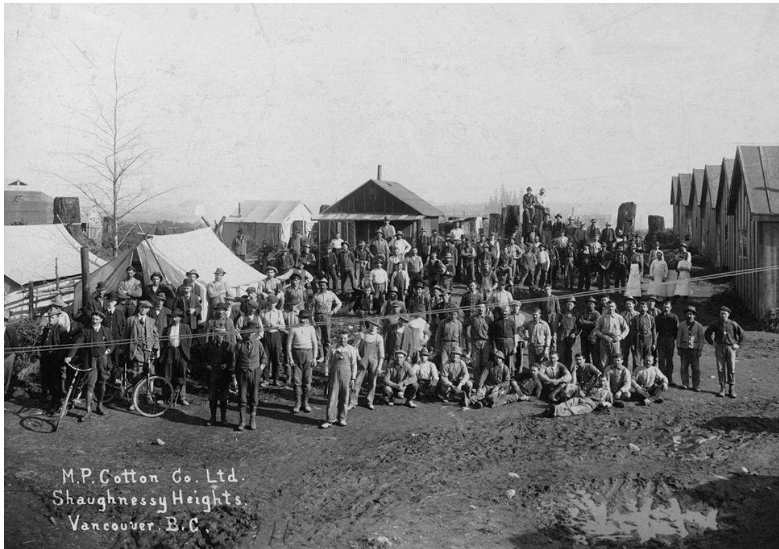
Figure 6 M.P. Cotton Co. Ltd. construction crew and carts in Shaughnessy Heights, 1911 [City of Vancouver Archives 677-249]
