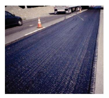
Tack coat using an asphalt emulsion. The black color indicates it has broken.
