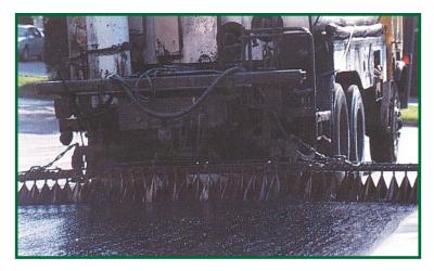
Set the height of the spray bar high enough above the roadway for the surface to receive double or triple coverage.
