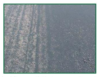
Poor (left) versus good (right) tack coat coverage. Note streaky coverage of poor coat and nearly complete coverage of good.
