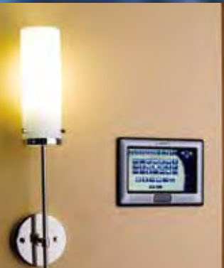
Above: One of several AMX panels used to control the audio and video throughout The Bravern.
