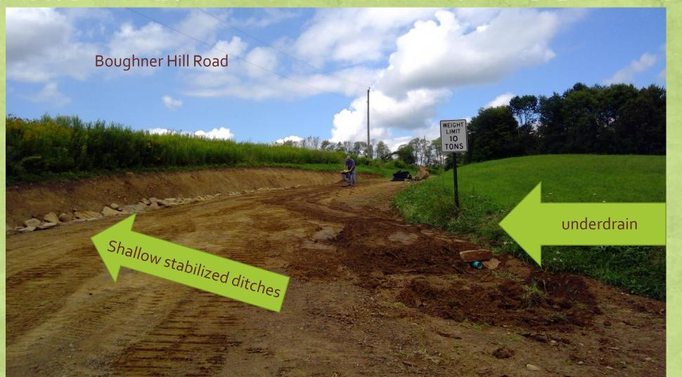
Stabilized ditches were constructed to carry stormwater from the cross pipes to pipes at the intersection.
