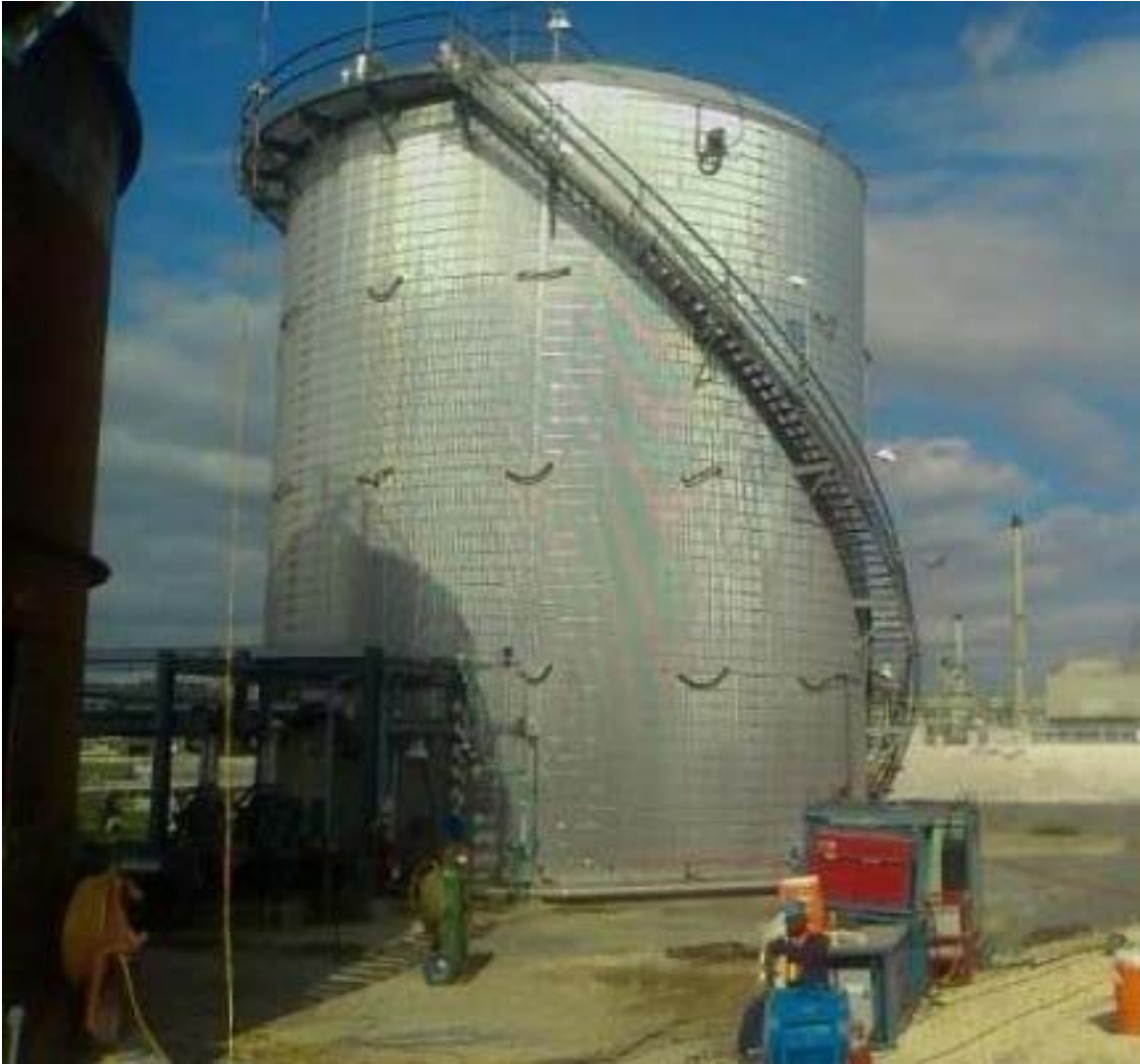
Figure 8: The tank completed in 2007
