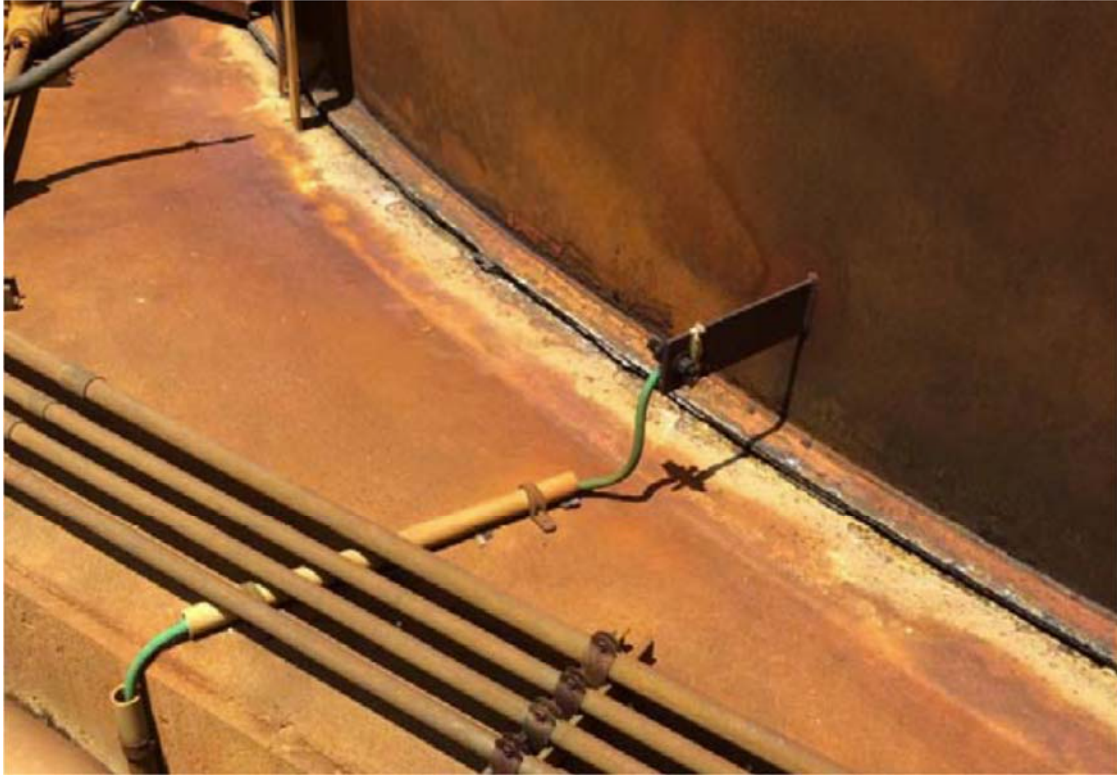
Figure 9: Tank chime overview (bottom corner)
