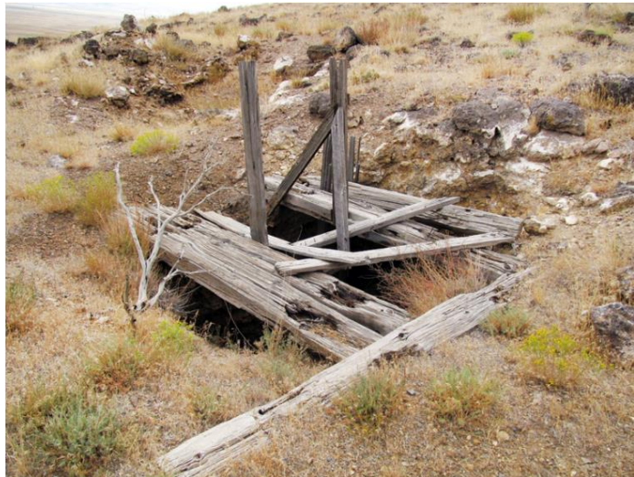
Abandoned workings on the San Francisco Mining District
