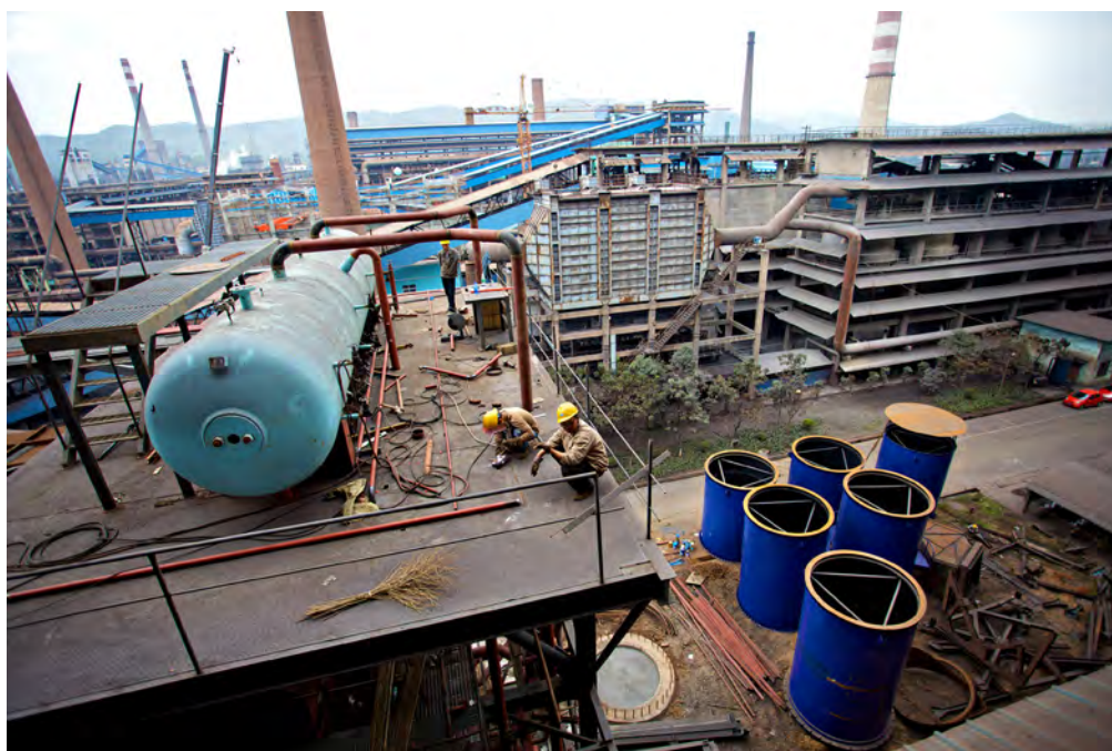
Workers conduct a massive retrofit of an iron plant to recapture previously wasted energy previously wasted in Guangdong, People's Republic of China.
