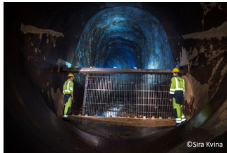
Trash rack in the Duge power plant
