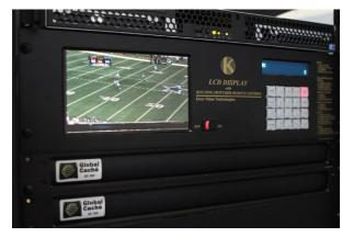
The remote keypad/LCD in the second-floor closet, where the sources are located, and the network interface.
