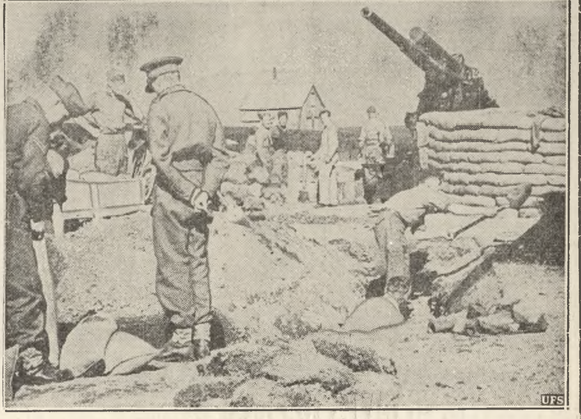
AMERICANS TAKE OVER—Uncle Sam's Marines have landed in Iceland for duration of war, to forestall German occupation of island and to assure delivery of American munitions to Britain. British formerly occupied island, as shown by these troops erecting gun emplacements at strategic points. Island is 2,500 miles from New York; 2,700 from Berlin.
