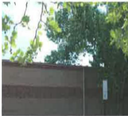
Limbs laying on roof
