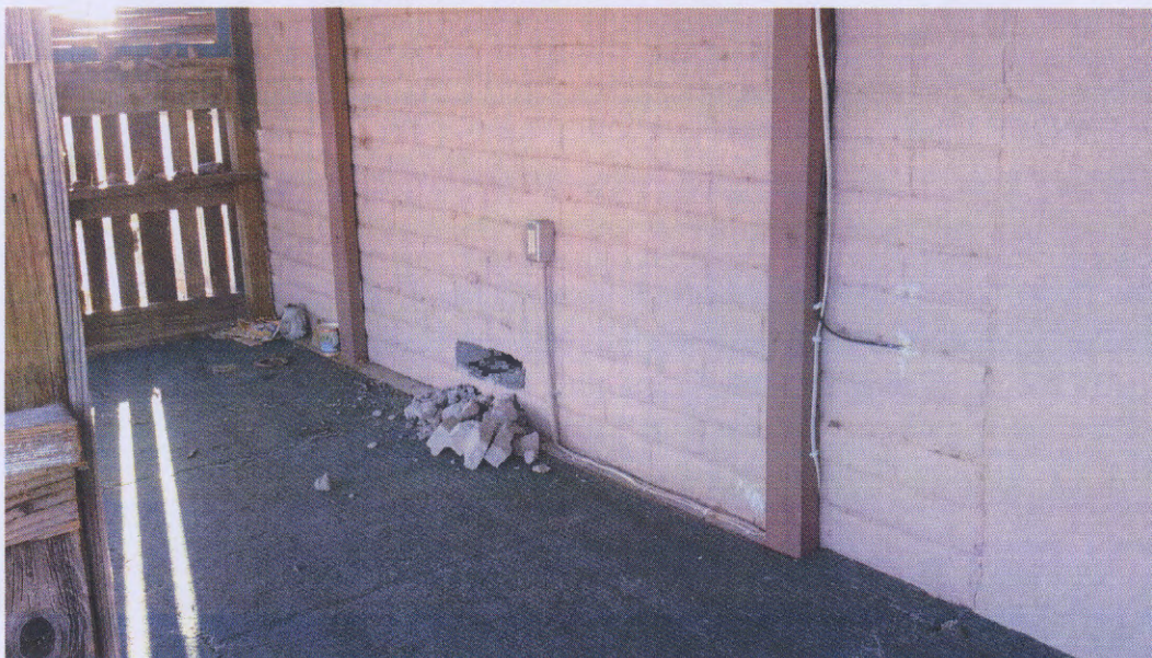
South Vent - Addition
