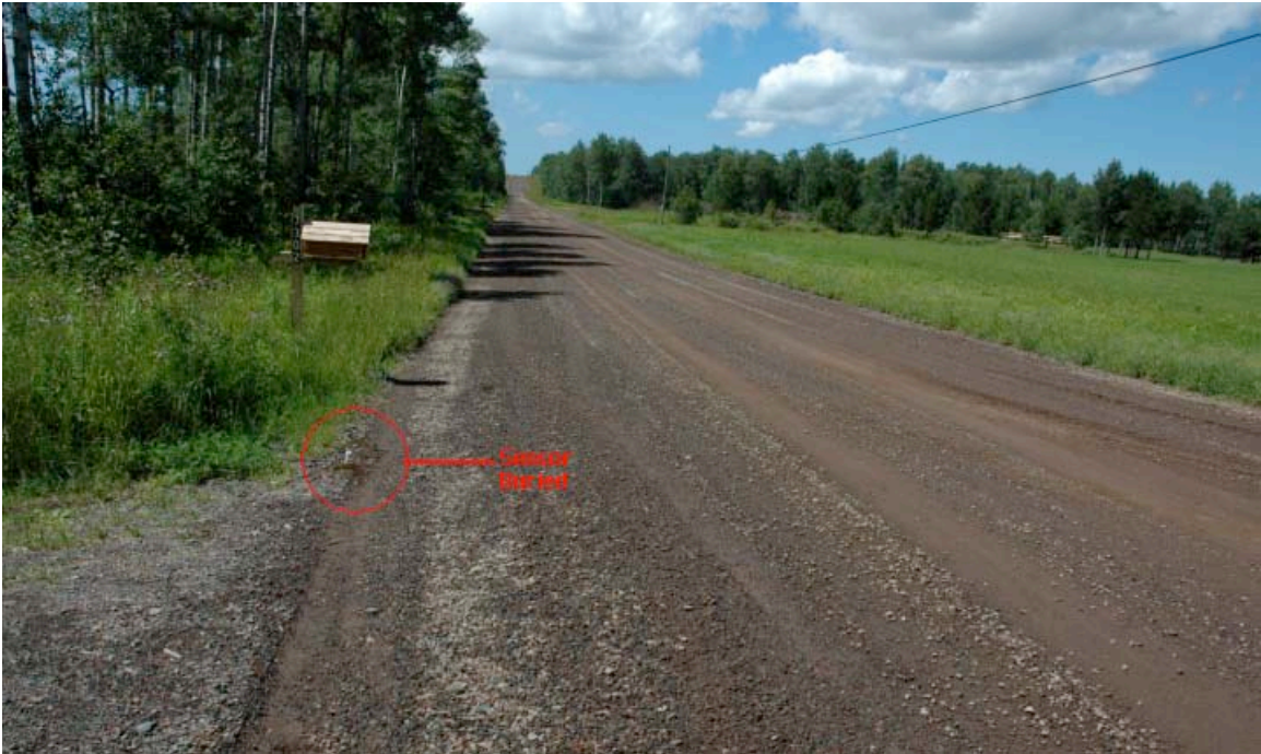
Figure 28: Sensor buried on the side of the road.
