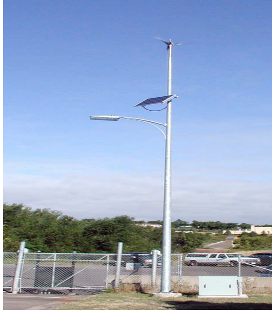
Figure 10: Completed Renewable Light Pole System.
