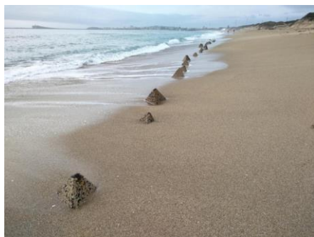
Erosion exposes remnants of WW2 defences along Newcastle's Stockton Beach. Source: Reddit .
