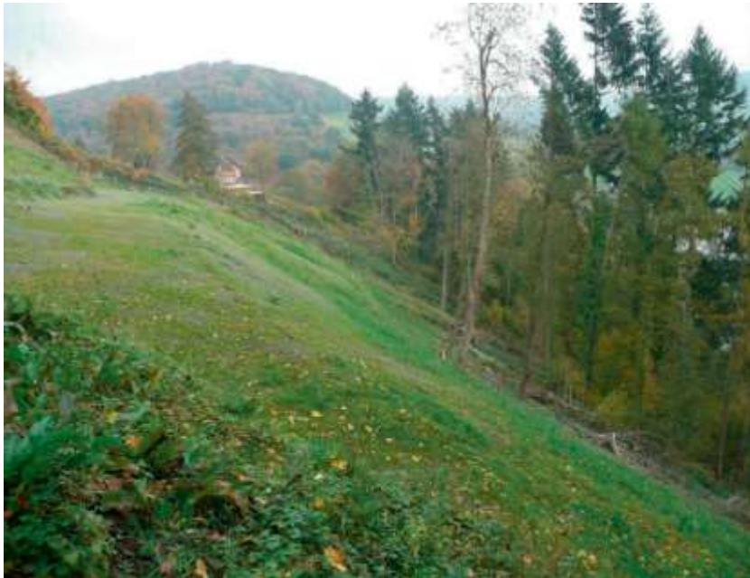
Picture 11.54 TECCO® system installed at Barbados Wood, Tintern, UK
