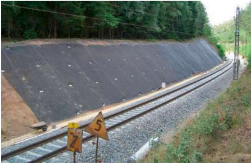
Picture 11.48 TECCO® system installed at Railway in Czech Republic
