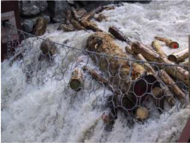
Picture 2.4 Example of driftwood protection barrier with ringnets made from high-tensile wires
