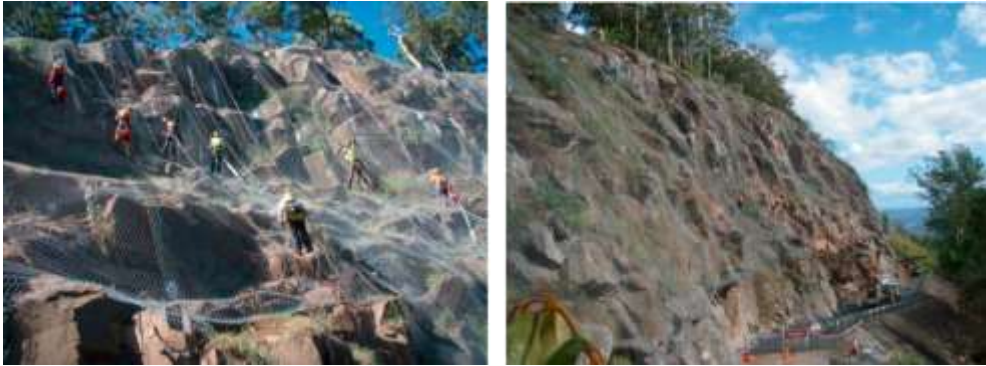
Picture 11.56 TECCO® installation at Mount Tambourine, Australia
