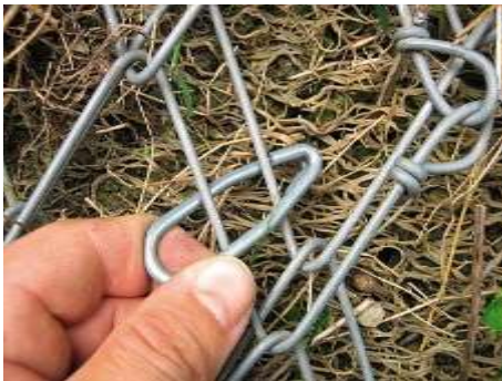
Picture 5.22 Hand application process for installation of connection clip
