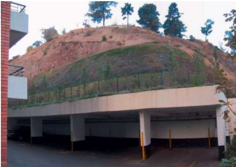
Picture 11.45 TECCO® system installed at La Luz, Santiago de Chile
