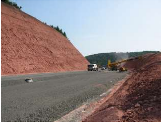
Picture 11.20 Situation before stabilizing
