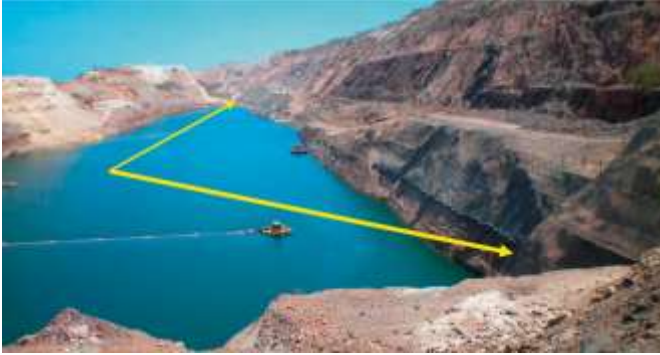
Picture 11.55 TECCO® installation at open pit mine in Western Australia
