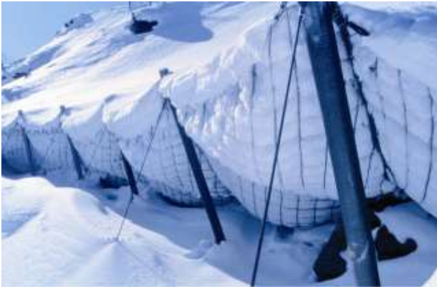
Picture 2.3 Example of avalanche prevention system made from rope wire nets
