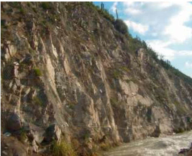
Picture 11.57 TECCO® installation at Puntilla Hydro Power Plant, Chile
