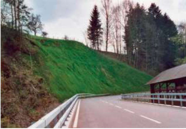
Picture 11.3 Completed slope stabilization system including greening (new bridge in front)
