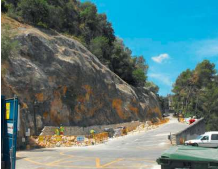
Picture 11.58 TECCO® installation at Xativa, Spain
