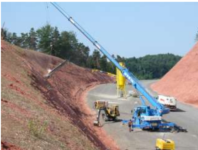
Picture 11.23 Drilling work using mobile cranes
