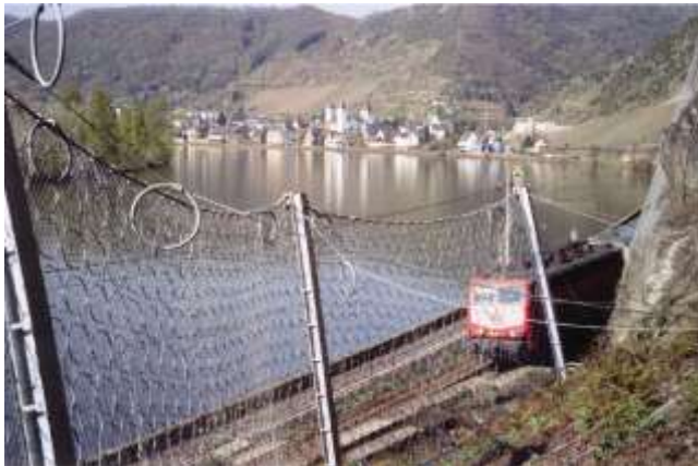
Picture 2.1 Example of rockfall barrier with ringnets made from high-tensile wires
