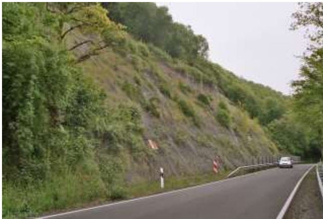
Picture 11.12 Overview stabilized area (several months after installation)
