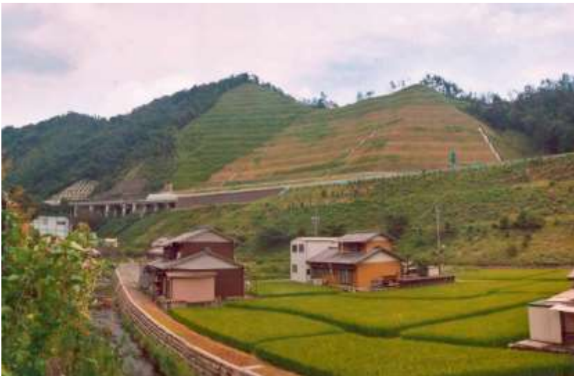
Picture 11.47 TECCO® system installed at Gifu Prefecture, Japan
