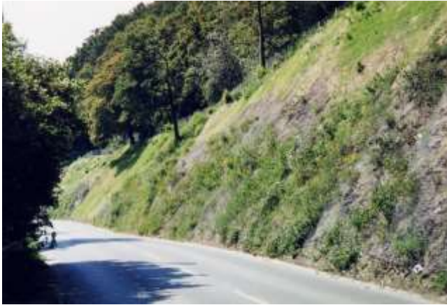
Picture 11.8 Completed installation with protected slope
