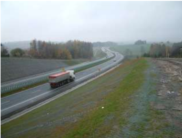
Picture 11.35 Completed slope after completion of Express Road works
