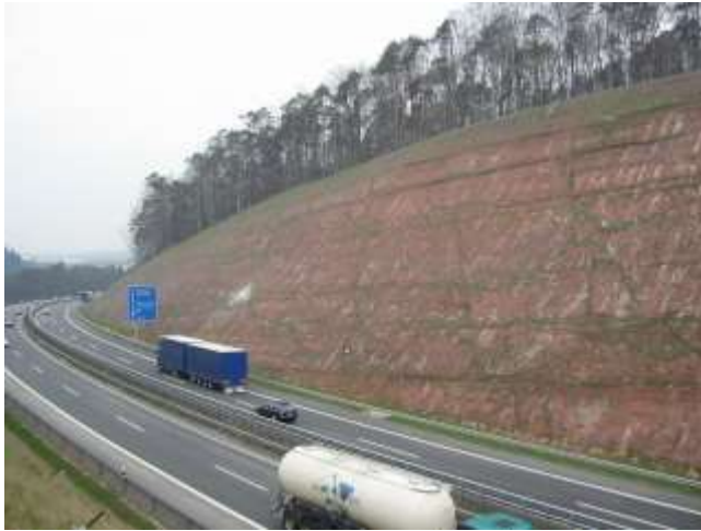
Picture 11.28 State of the stabilized slope several months after installation
