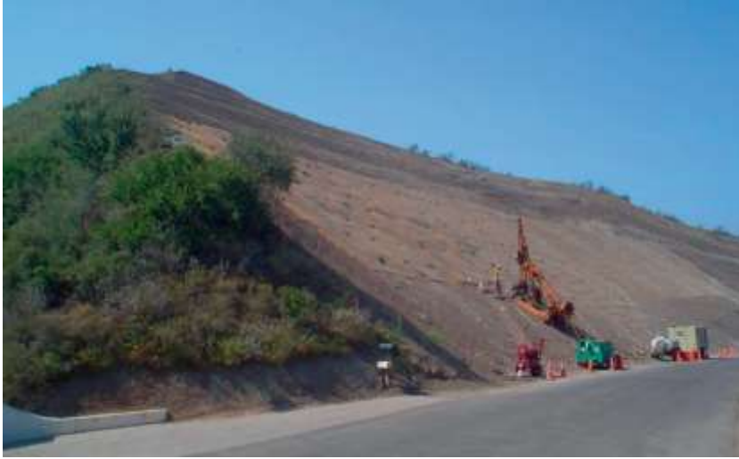
Picture 11.44 TECCO® system installation at Santa Barbara, USA (under construction)
