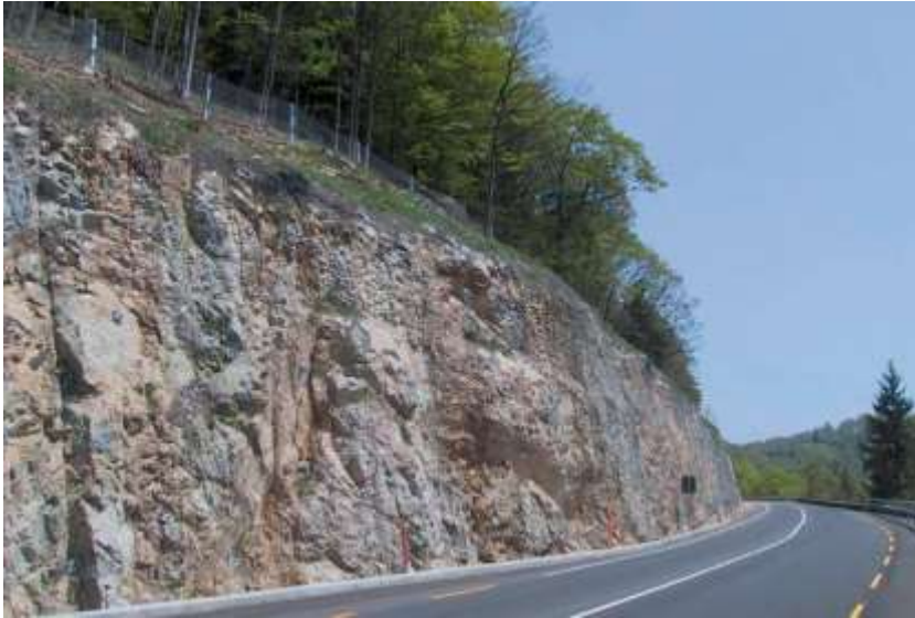
Picture 11.40 TECCO® system installed at Brot-Dessous, Rochefort, Switzerland
