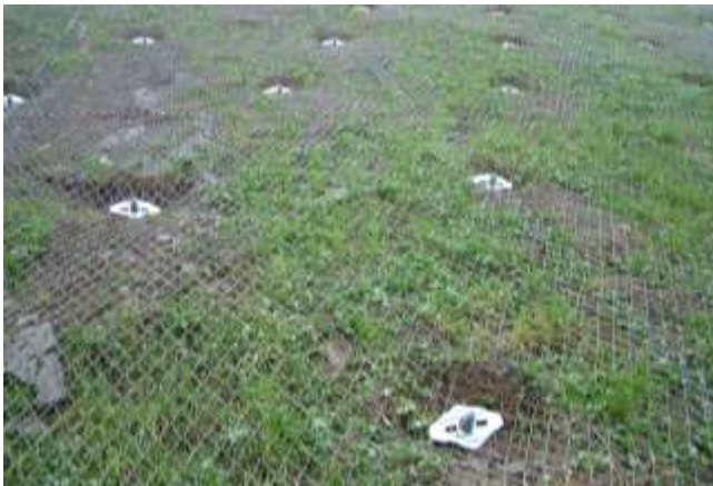
Picture 11.33 System spike plates allow active pretensioning (system fully installed)
