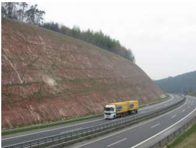
Picture 11.29 State of the stabilized north-western slope several months after installation
