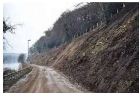
Picture 10.5 Left: Slope during preparation measures (clearing, levelling, partial cutting, etc.) Right: Slope after preparation measures
