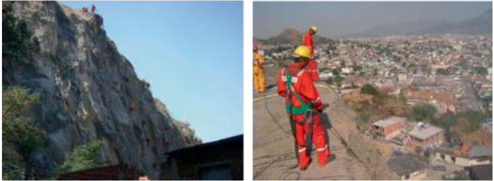
Picture 11.53 TECCO® system installation at Cavalcanti, Rio de Janeiro, Brazil
