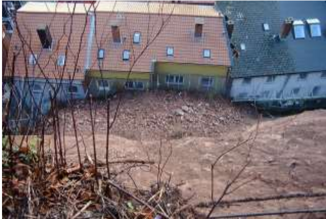
Picture 11.15 Sliding mass at the foot of the slope
