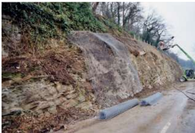
Picture 10.12 Unrolling of the mesh before installation of the nails
