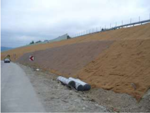
Picture 11.38 Slope covered with cocomat during high-tensile steel wire mesh installation
