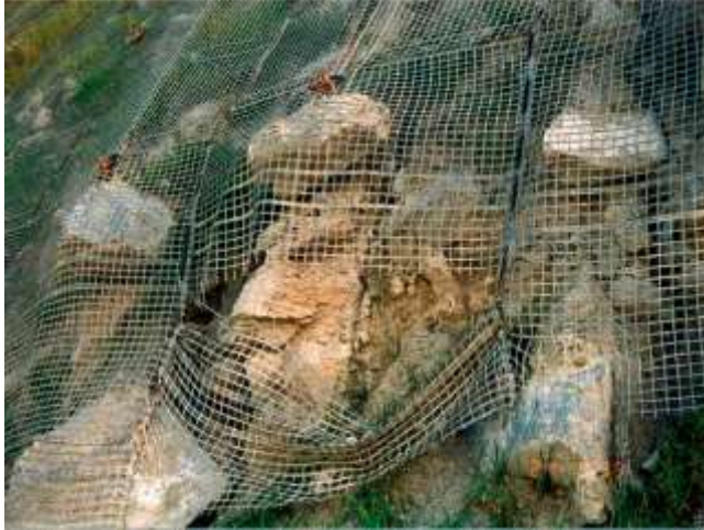
Picture 3.4 Soft facing (sample for high-tensile geogrid)
