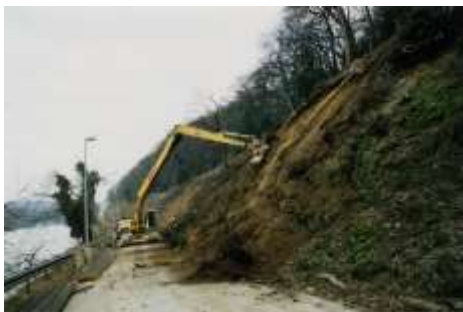
Picture 10.5 Left: Slope during preparation measures (clearing, levelling, partial cutting, etc.) Right: Slope after preparation measures
