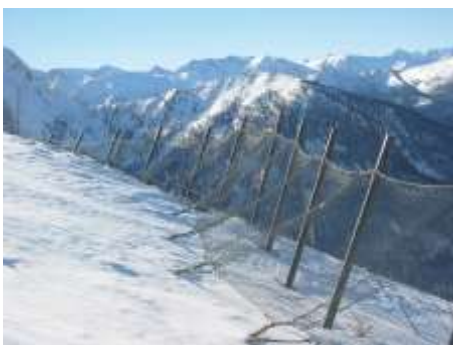
Picture 5.2 Avalanche prevention system with high-tensile steel wire mesh
