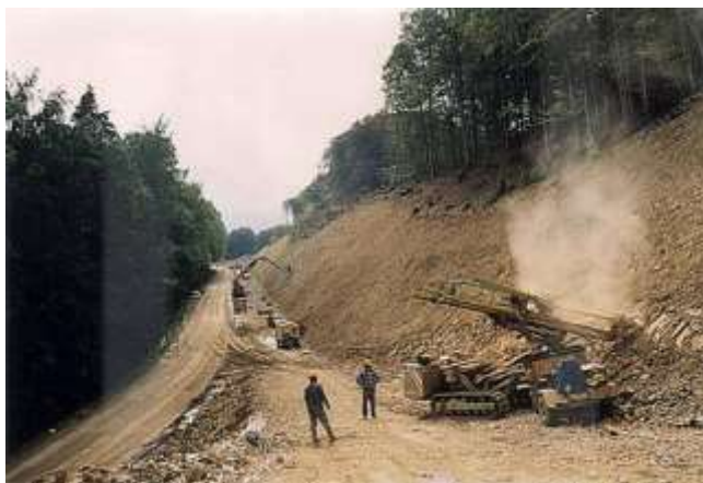
Picture 10.10 Drilling work using a crawler-mounted drilling device (dry drilling)
