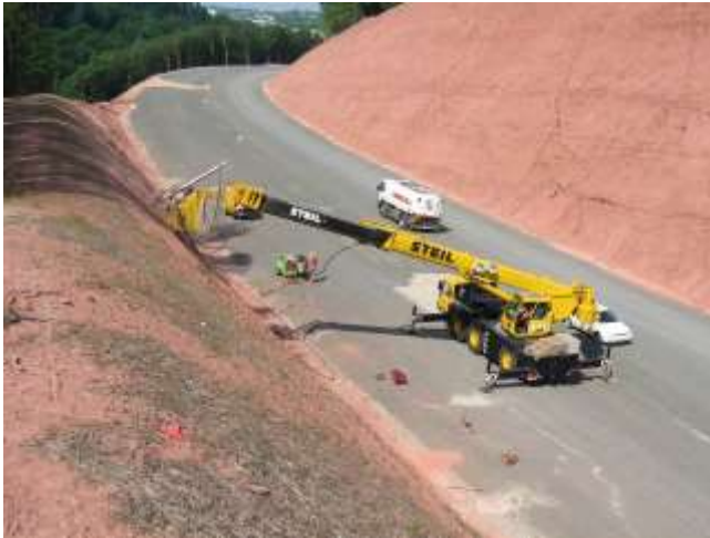
Picture 11.22 South-eastern slope: drilling work
