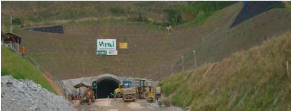
Picture 11.51 TECCO® system installed at Tunnel do Morro Agudo, Brazil
