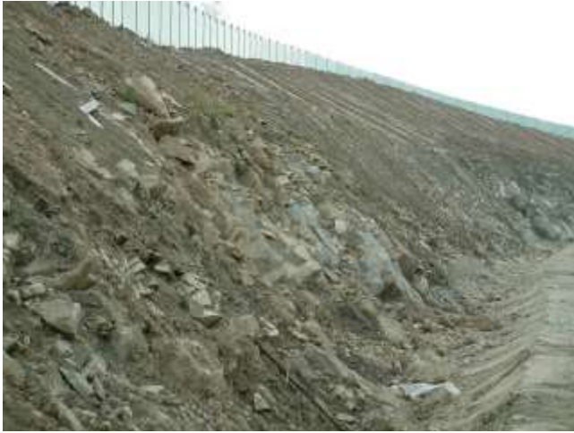
Picture 11.36 Rough slope after cutting; the drainage system is visible at the upper part of the slope over the bench
