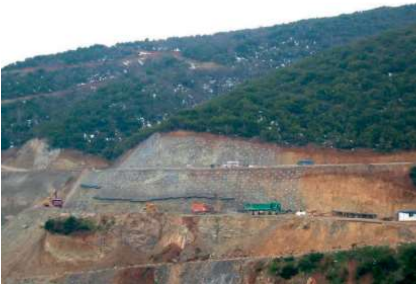
Picture 11.43 TECCO® system installation at Polymilou, Greece (under construction)
