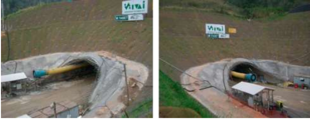
Picture 11.50 TECCO® system installed at Tunnel do Morro Agudo, Brazil
