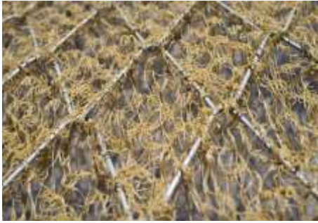
Picture 8.2 Erosion control mat integrated with high-tensile steel wire mesh
