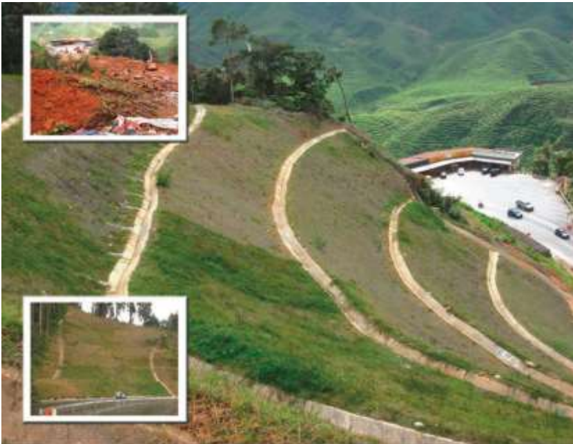
Picture 11.61 TECCO® installation in Malaysia
