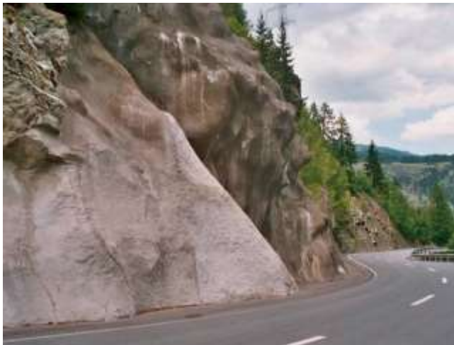
Picture 3.1 Hard facing (sample for shotcrete slope stabilization system)
