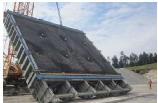
Picture 13.5 Test no.11, TECCO® G65/3 + P33, nail grid 3.5 x 3.5 m, sandy gravel 0 – 63 mm, \alpha = 53^\circ , first slides close to the surface
