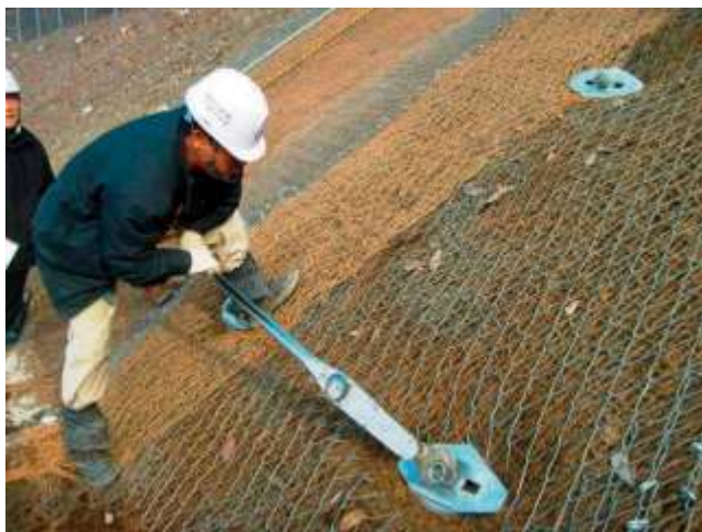
Picture 10.15 Pretensioning of spike plates
