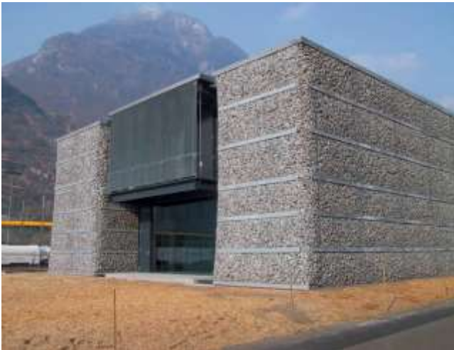
Picture 11.68 Special TECCO® application at Alptransit exhibition centre, Bodio, Switzerland
