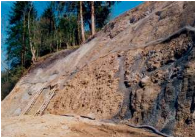
Picture 11.2 Drainage measurements before mounting of the TECCO® mesh
