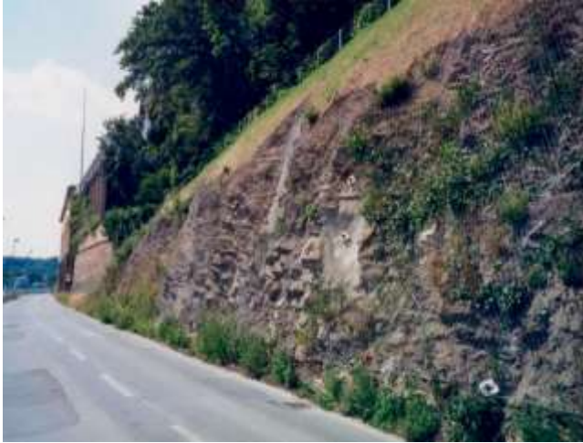
Picture 3.2 Flexible facing (slope stabilization system with high-tensile steel wire mesh)
