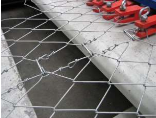
Picture 5.27 Condition right after the collapse of the high-tensile steel wire mesh
