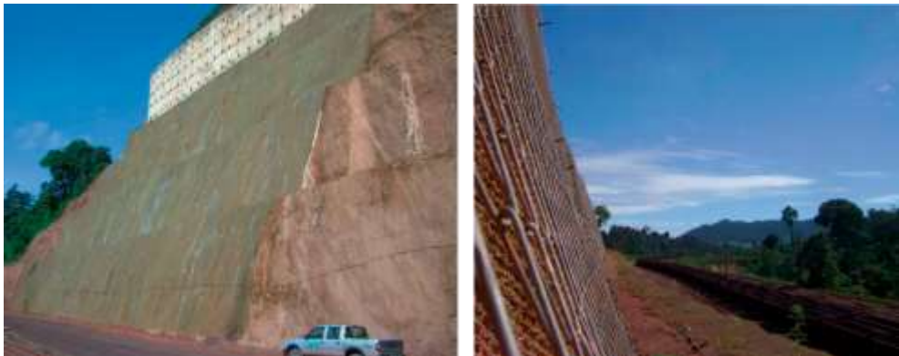
Picture 11.52 TECCO® slope stabilization at Carajas in Brazil (for VALE)
