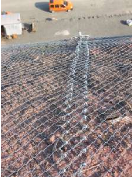
Picture 11.27 Connection of mesh panels
