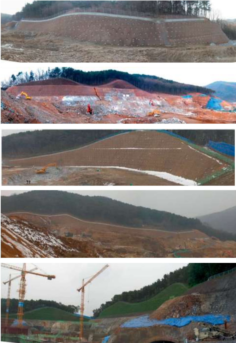
Picture 11.62 TECCO® slope stabilizations incl. greening for SAMSUNG in Korea
