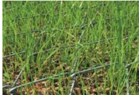
Picture 8.1 TECMAT Erosion control mat installed underneath the TECCO® mesh
