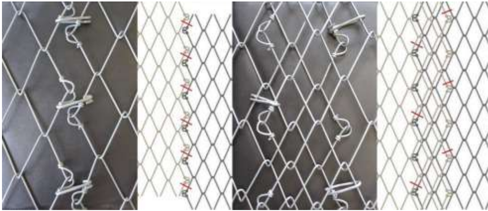
Figure 10.6 Left: Connection without overlap for TECCO® G45/2 and TECCO® G65/3 Right: Connection with overlap of 2 diamond mesh units for TECCO® G45/2 and TECCO® G65/3
