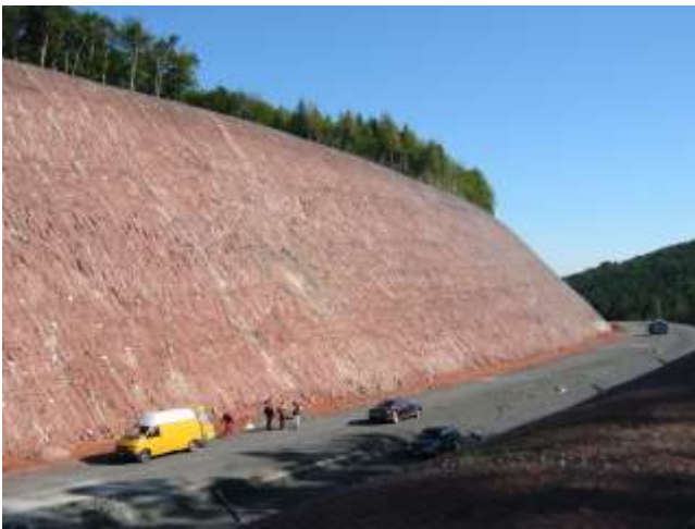
Picture 11.25 Stabilized slope
