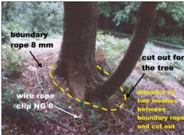
Picture 10.20 Example for tree hole installation
