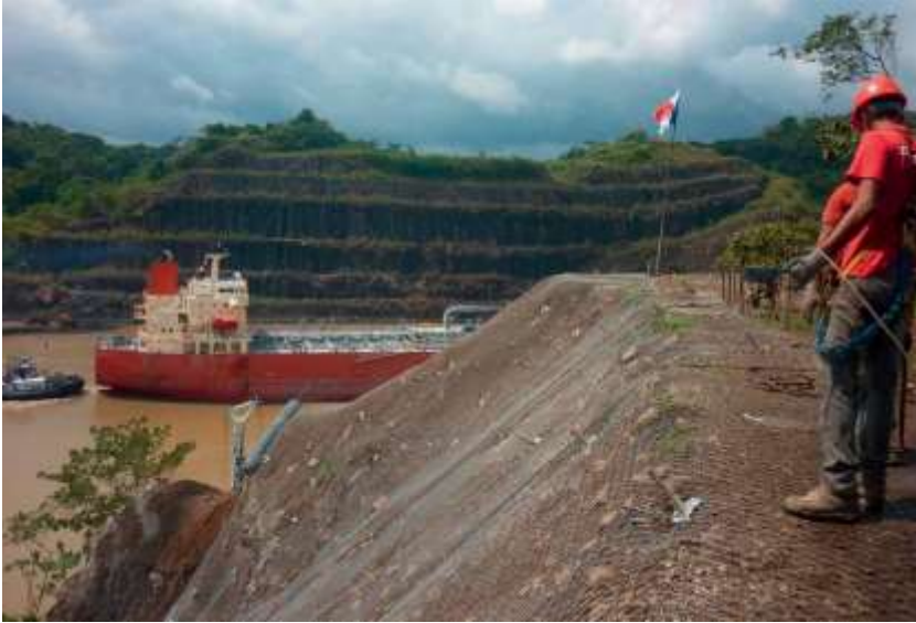
Picture 11.60 TECCO® installed at the Panama Channel, Panama
