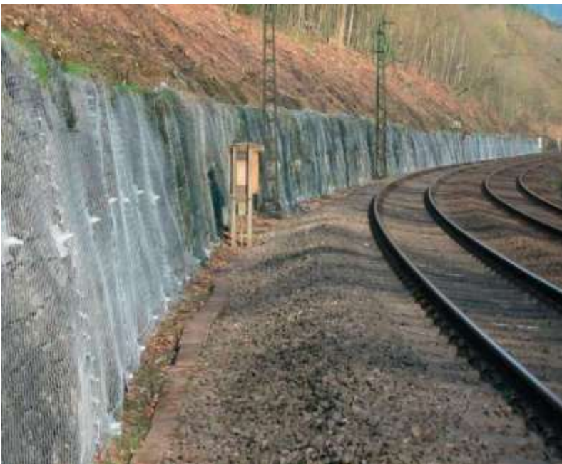
Picture 11.66 Stabilized brick wall (covered and nailed with TECCO® mesh)
