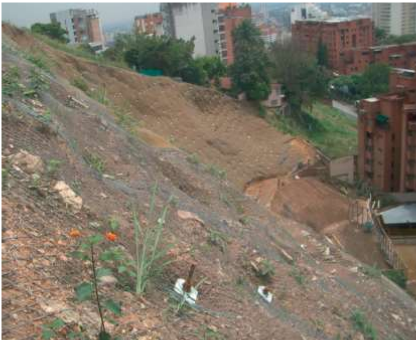
Picture 11.59 TECCO® installation at Monte Rosa Cali, Colombia
