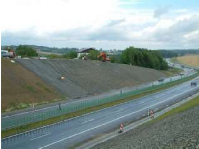
Picture 11.32 Installation of the high-tensile steel wire mesh
