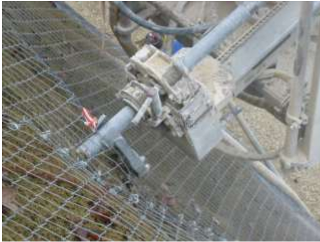
Picture 10.9 Detail of drilling process using the drilling tool
