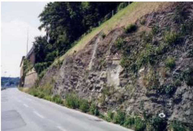
Picture 11.9 Completed installation with protected slope (rocky section)
