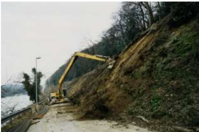
Picture 11.5 Cleaning and natural grading with excavator
