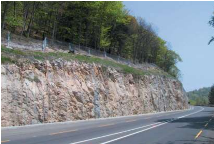
Picture 11.41 TECCO® system installed at Brot-Dessous, Rochefort, Switzerland
