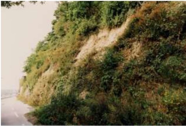
Picture 11.4 View of the slope and sliding areas before installation
