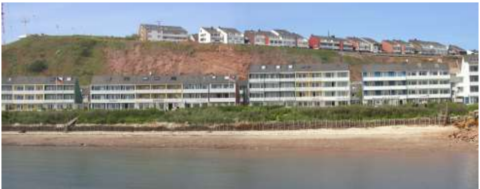
Picture 11.19 Overview of the slope stabilization of the Falm edge of Helgoland (Germany)
