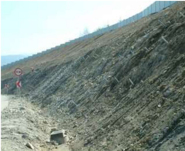
Picture 11.37 Reprofiled and nailed slope face
