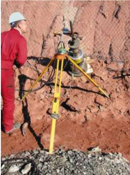
Picture 11.26 Pulling tests
