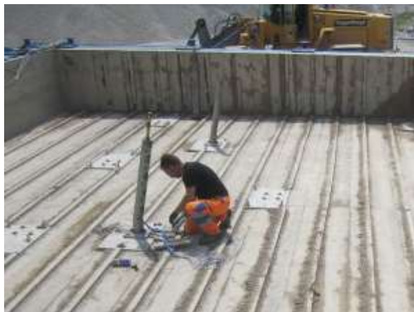
Picture 13.1 Test no. 13, TECCO® G65/4 + P33, after dismantling mesh cover and removing material, nail grid 3.5 x 3.5 m
