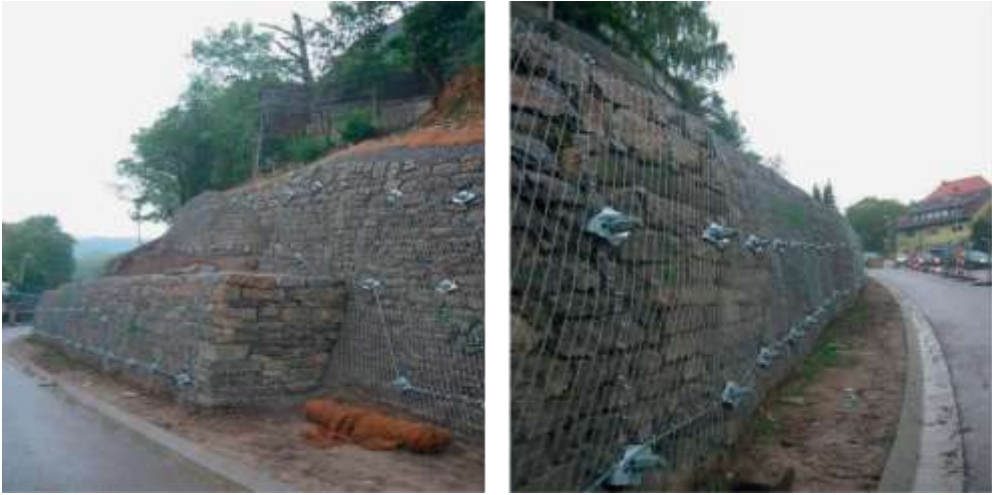
Picture 11.67 TECCO® stabilization of brick walls at Markgröningen, Germany
