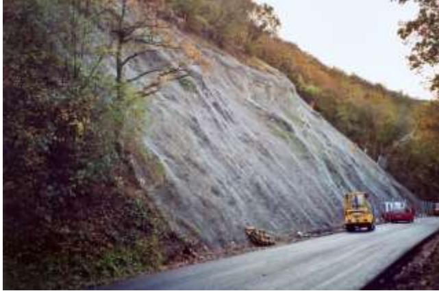
Picture 11.11 Overview stabilized area (after completion of installation work)
