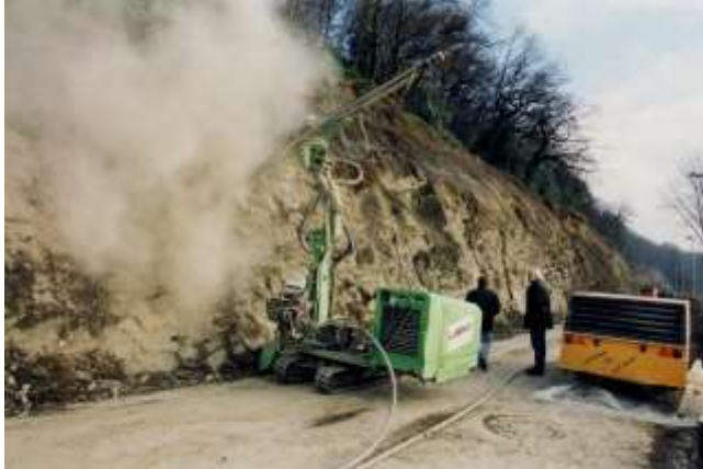
Picture 11.6 Drilling process
