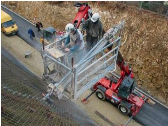
Picture 10.8 Drilling process from crane basquet using the drilling tool
