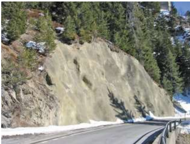
Picture 10.21 Slope stabilization using traditional reinforced shotcrete system
