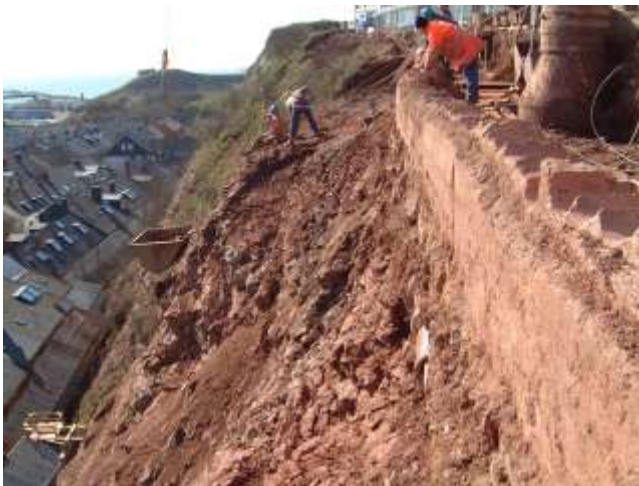
Picture 11.16 Cleaning work
