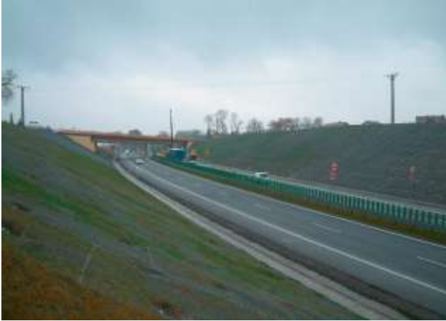
Picture 11.34 Slopes after completion. Slope partially covered with crushed stones, no greening was applied and no erosion mat was used
