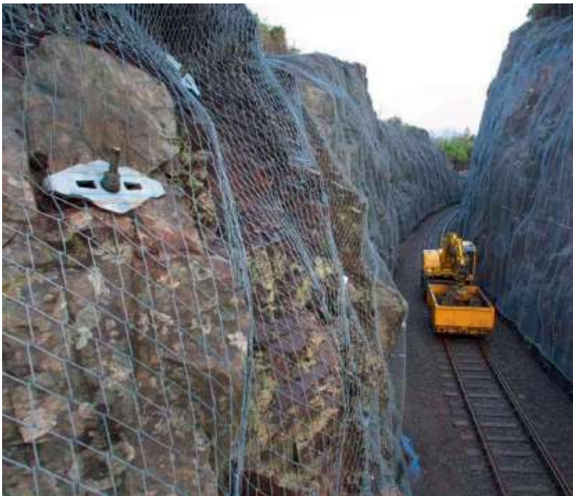
Picture 11.49 TECCO® system installed for railway protection at Kyle, UK
