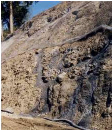
Picture 10.17 Filter drain filled with concrete to drain arising hillside water
