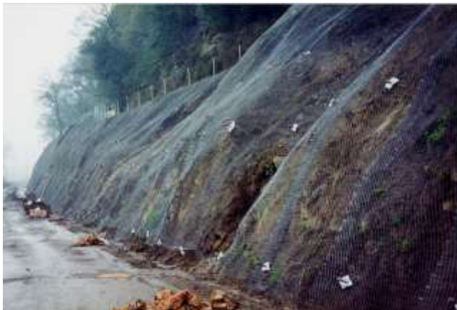
Picture 11.7 Installation of high-tensile steel wire mesh
