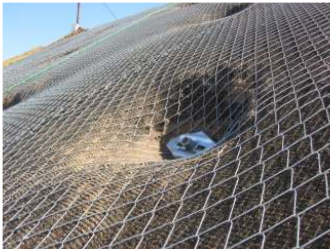
Picture 10.13 Positioning of spike plates
