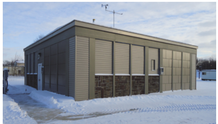
Wall Assembly Research Center: A laboratory built by The Dow Chemical Company in Midland, Michigan to test the performance of several different wall assemblies in real world conditions.
