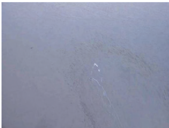
Figure 5. Photos show examples of Class III leak
