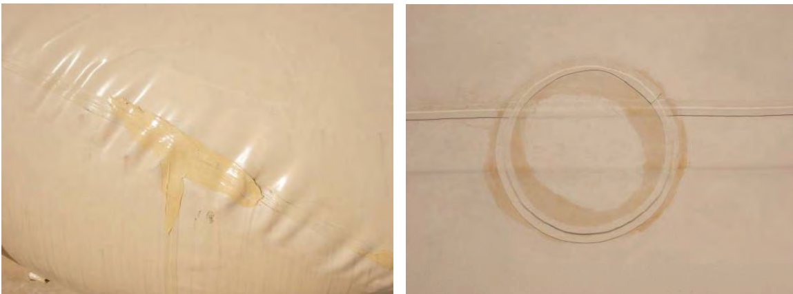
Figure 1. Two examples of manufacturer repairs/patches not considered deficiencies during the baseline inspection.
