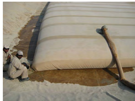
Figure 5. Photos show examples of Class III leak
