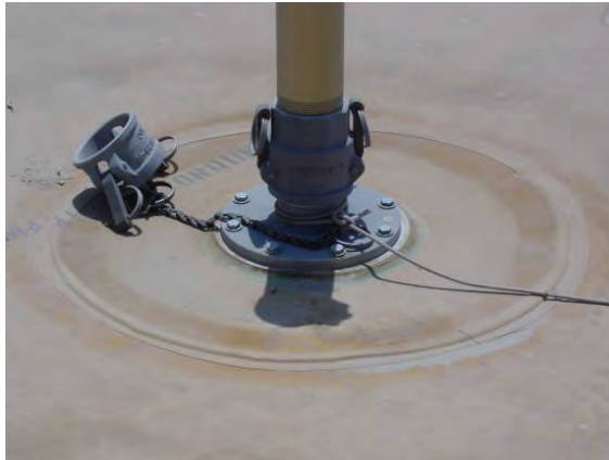
Figure 19. String secured to vent.
