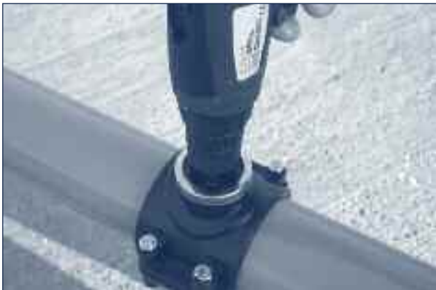
④ Drill a hole in the pipe taking care not to damage the reverse of the pipe or the gasket.
