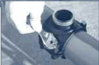
③ Couple the bottom part of the saddle with the upper one. Insert the bolts from the bottom, screw the nuts and tighten the bolts diagonally opposite each other.
