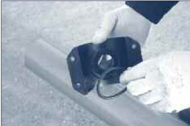
② Put the O-ring in the relevant seat and position the upper part of the saddle on the pipe.
