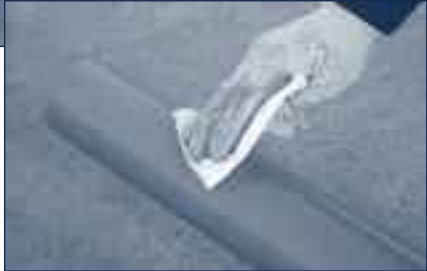
① Define the position of the branch and clean the external surface of the pipe.
