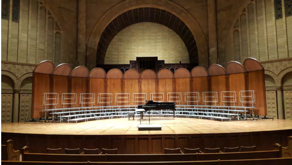
The 13-piece acoustical shell helps performers onstage hear each other and clarifies sound for the audience
