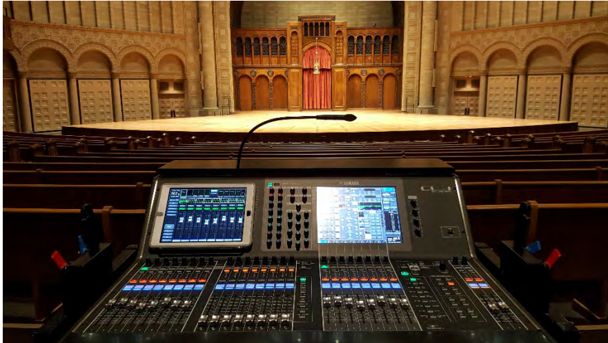
View from the Front of House overlooking the Yamaha CL3 mixing console
